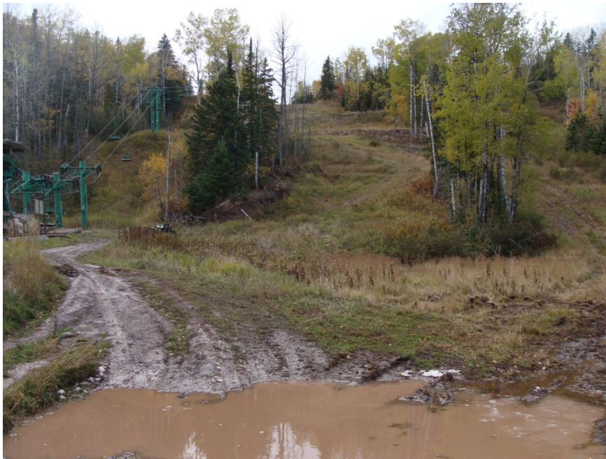
Figure 26. Ponded area at base of ski slopes with direct access to river
