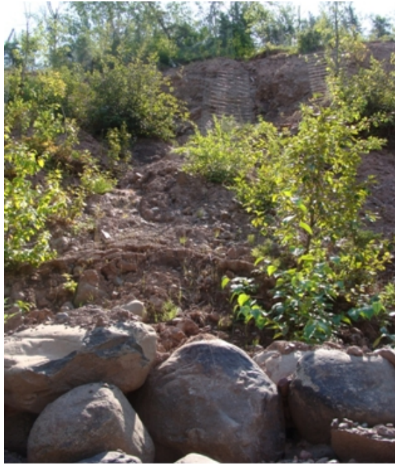
Figure 9. Shows sediment deposited down slope, on top of the boulders which were placed to reduce toe erosion. This sediment will be transported down stream during the next high flow event.
