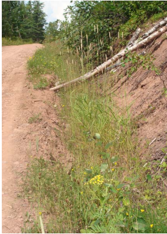
Figure 6. Shallow ditch and road cut
