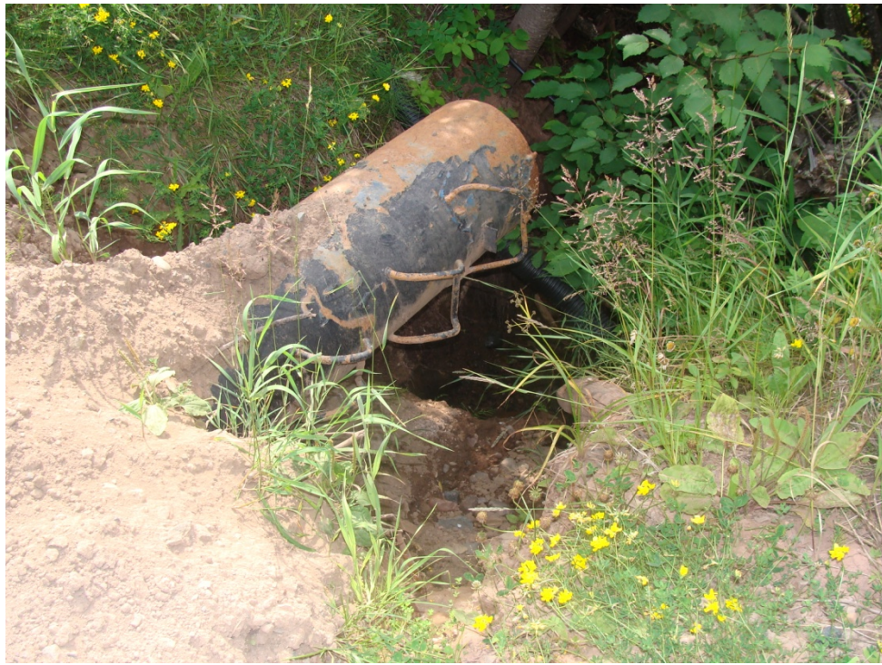
Figure 21. Perched culvert.
