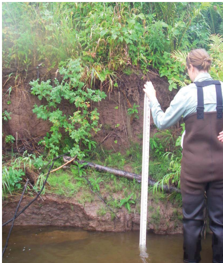
Figure 58. Stream bank in an old lake bed C4 channel (the BR5 site).
