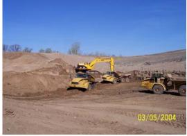
Subgrade excavationn for cell construction at the Elk River Landfill.
