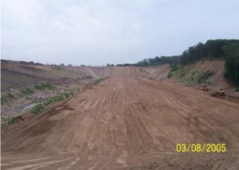
Sand drainage layer in completed cell at Elk River Landfill.
