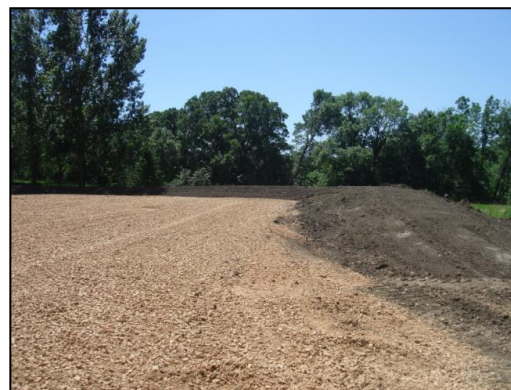
Above: Gravel covering active composting areas of site.
