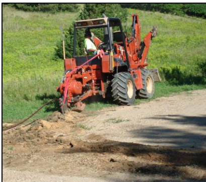
Above (left): Minnesota Valley Electrical Cooperative trenches cable along the service road of the site.
