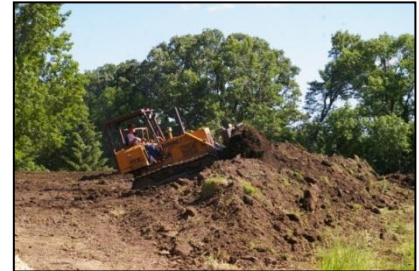
Above: Visual berm being constructed. Below: Laying seed and hay on visual berm.
