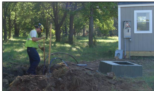
Above (left): Minnesota Valley Electrical Cooperative trenches cable along the service road of the site.
