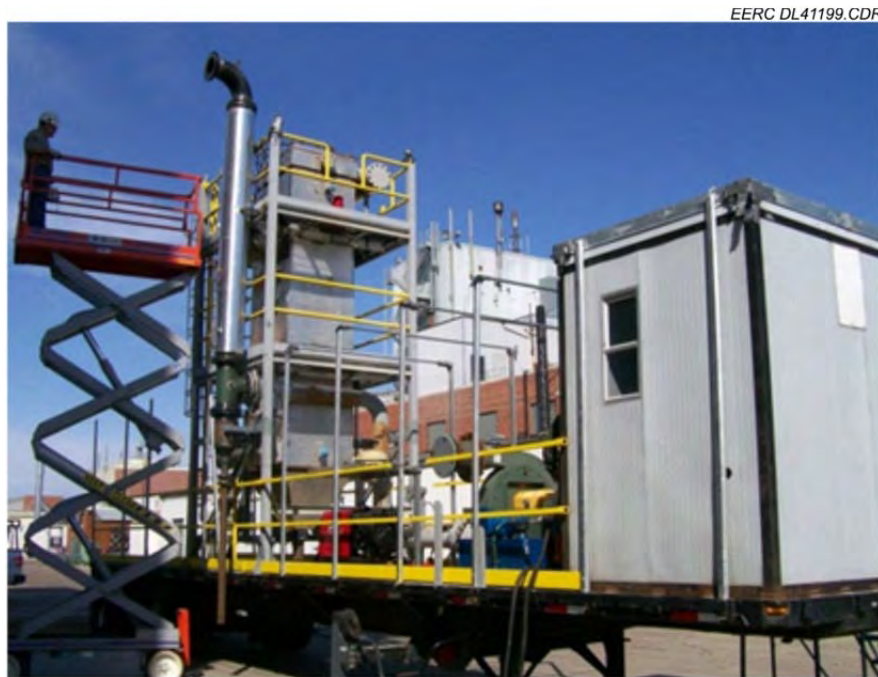
Figure ES-1. Baghouse, trailer, and control room.
