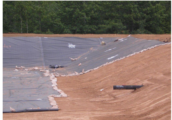
Figure 8-10: Installing a synthetic liner
