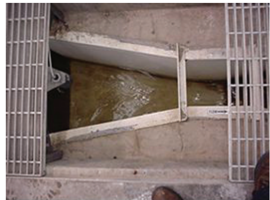
Figure 3-2: Parshall flume
