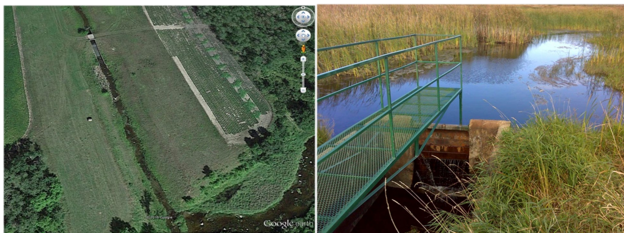
Figure 53. Photos of connectivity barriers along AUID 514, including a grade control structure on September 1, 2013, courtesy of Google Earth (left), and the Horseshoe Lake Dam on September 23, 2015 (right).
