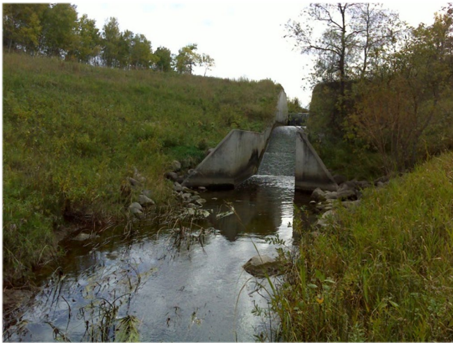
Figure 86. Photo of a grade control structure along AUID 549, near its confluence with the North Branch Two Rivers, on September 30, 2015.
