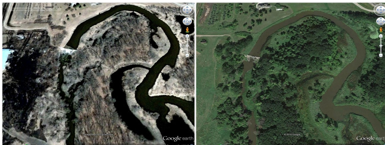
Figure 47. Photos of the Northcote Dam along AUID 508 on April 18, 2007 (left) and September 1, 2013 (right), courtesy of Google Earth.
