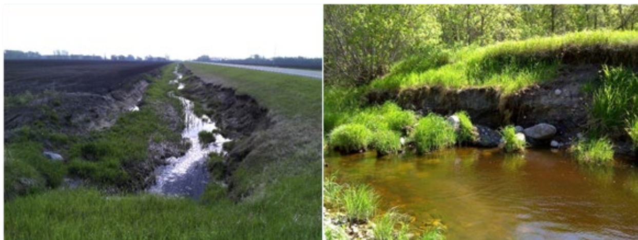
Figure 8. Images of sediment sources to AUID 543, including bank slumping along an unnamed ditch at the 200 th Avenue NW and CSAH 14 intersection on May 28, 2014 (left), courtesy of Clark and Vinje (2017); and bank erosion near Station 13RD104 on May 29, 2014 (right), courtesy of Clark and Vinje (2017).
