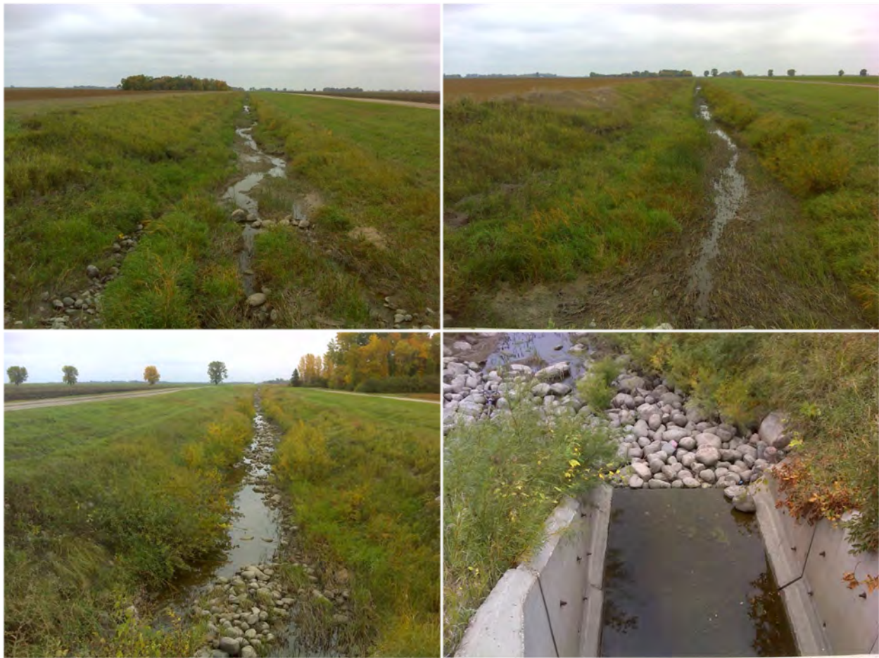
Figure 13. Photos of intermittent flow conditions along AUID 515 on September 24, 2014, including the 360 th Avenue NW crossing (upper left), the 370 th Avenue NW crossing (upper right), the 380 th Avenue NW crossing (lower left), and the 440 th Avenue NW (lower right).
