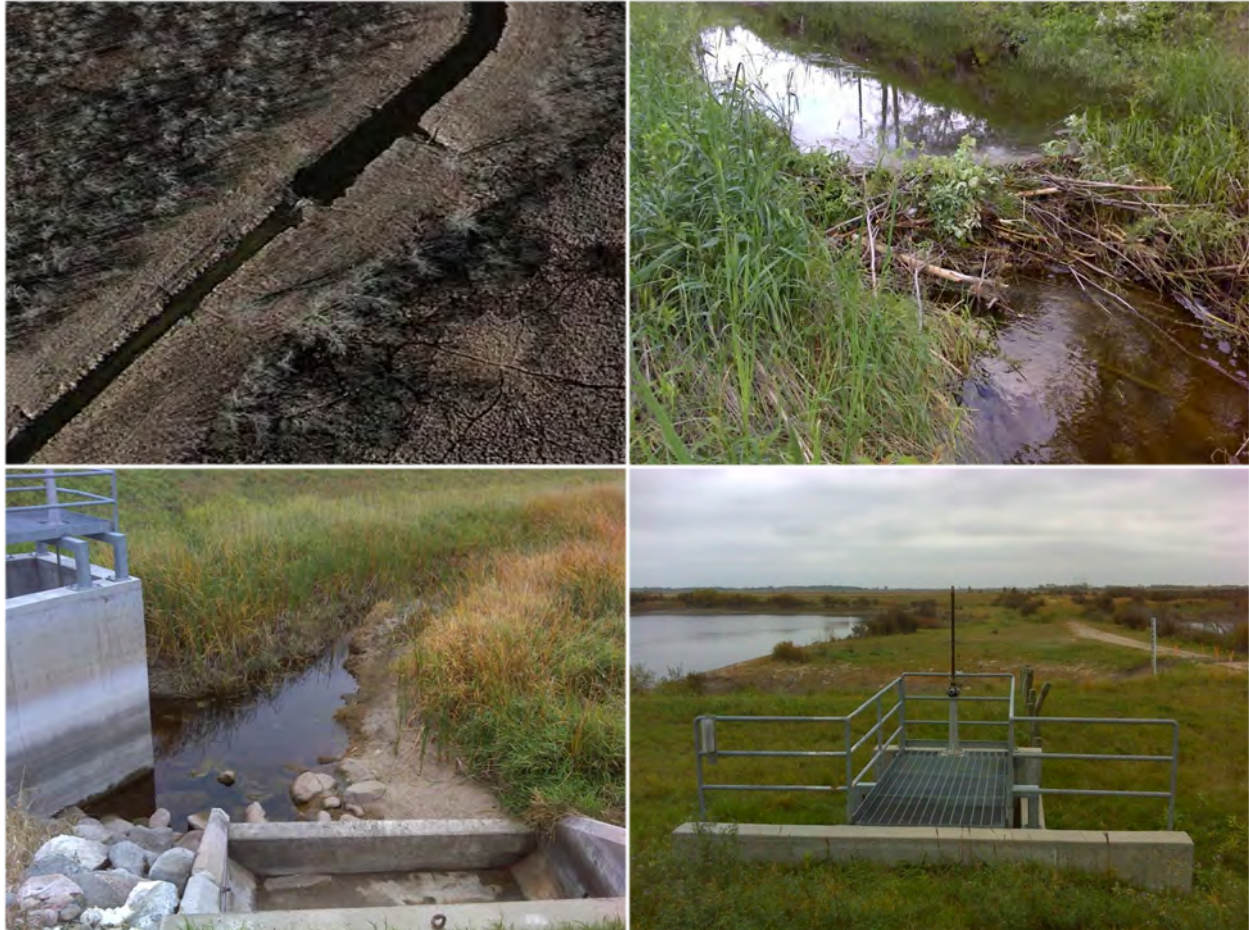
Figure 20. Photos of connectivity barriers along AUID 517, including a beaver dam immediately upstream of Site S008-175 on April 2, 2012, courtesy of Google Earth (upper left); a beaver dam immediately downstream of Site S008-175 on July 2, 2014 (upper right); the inlet structure of the Angus-Oslo #4 Impoundment on September 24, 2014 (lower left); and the outlet structure of the Angus-Oslo #4 Impoundment on September 24, 2014 (lower right).
