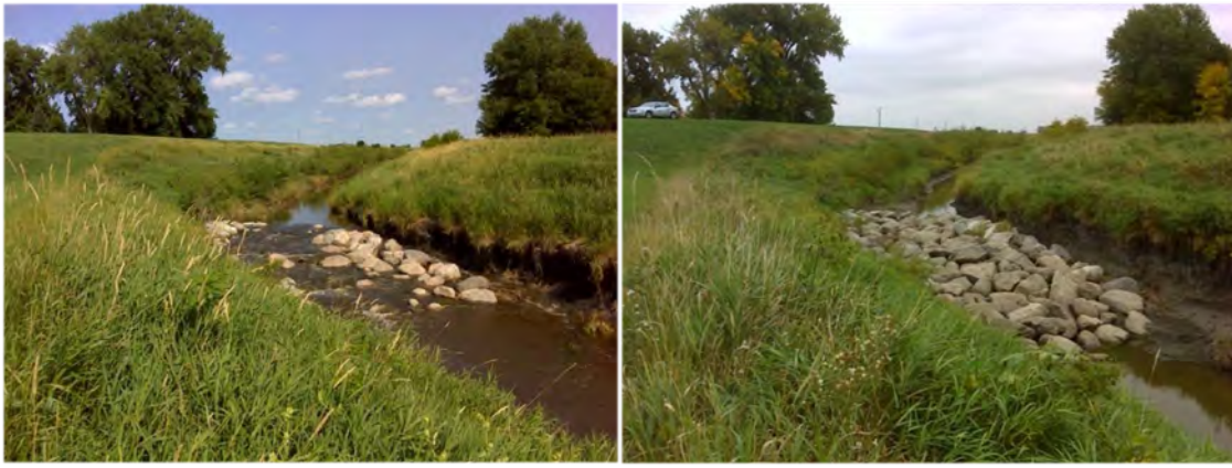
Figure 8. Photos of a rock check dam along AUID 515 immediately upstream of its confluence with the Grand Marais Creek on July 30, 2014 (left) and September 24, 2014 (right).
