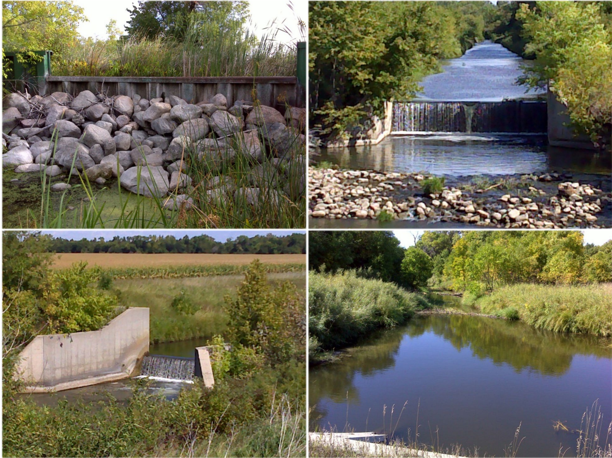
Figure 5. Photos of connectivity barriers along Reaches 541 and 542, including the Sand Hill Lake outlet dam (upper left), grade control structures (upper right and lower left), and a beaver dam (lower right)
