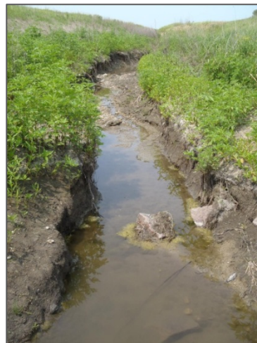
Photo 7. This ditch has incised and clearly contributes sediment to the South Fork Rabbit River, which it meets right at the bottom of this photo.
