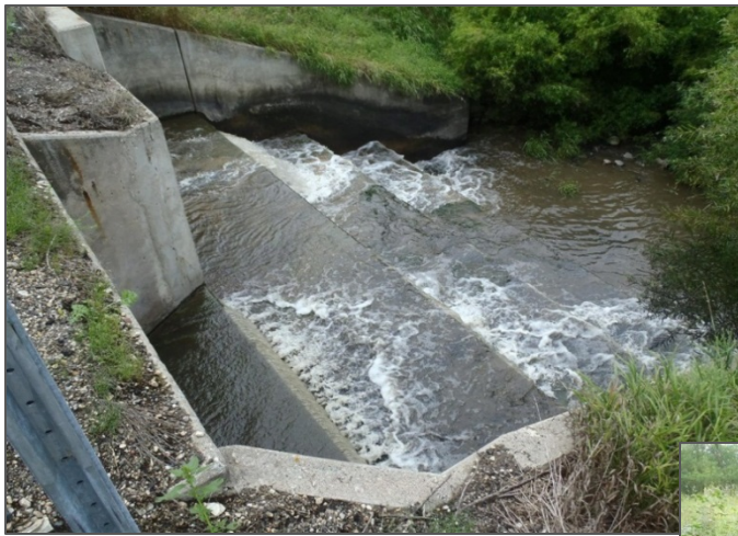
Photo 24. The culvert outlet at the Township Road 18 crossing is elevated by about two feet above the stream water level.
