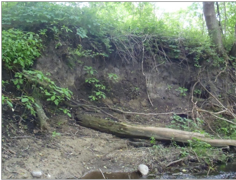
Photo 16. This badly-eroded bank, just upstream of State Highway 27, is evidence of channel instability. The top of the bank is about seven to eight feet above the water level in the photo.
