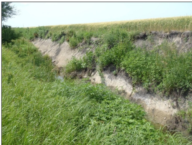
Photo 6. A ditch that is too narrow and deep to be stable. Clods of soil are falling down from the field edge, contributing topsoil into the ditch that will be washed into streams. There is also no buffer along this field edge.
