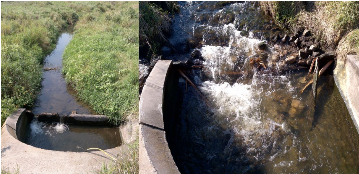
Figure 16: Fish barrier on AUID 503 (left). This barrier was documented in 2015, and was blown out (right) during a high flow event sometime late summer/early fall of 2016.
