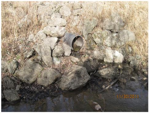
Figure 10: Example of a drain tile outlet to a stream in the Cedar River Watershed.
