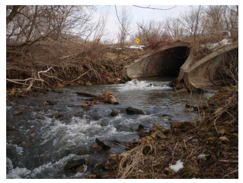
Figure 65. Perched culvert at CR17 and Station 08LM018. MPCA photograph March 18, 2011.
