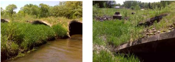
Figure 131. Culverts that have been partially filled with sediment at Site 12LM077 along Badger Run.
