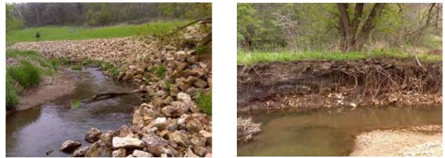
Figure 25. Left: Rip-Rap near biological station 12LM018. Right: Raw bank downstream of 12LM018, both photos demonstrating instability and erosion within the upstream area.
