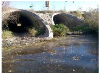
Figure 146. Backed up flow (MPCA photo 2015) on upstream end of culverts at CR22/Cascade Creek intersection
