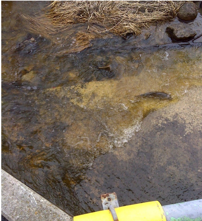
Figure 229. Fish swimming upstream through culvert on May 28, 2013
