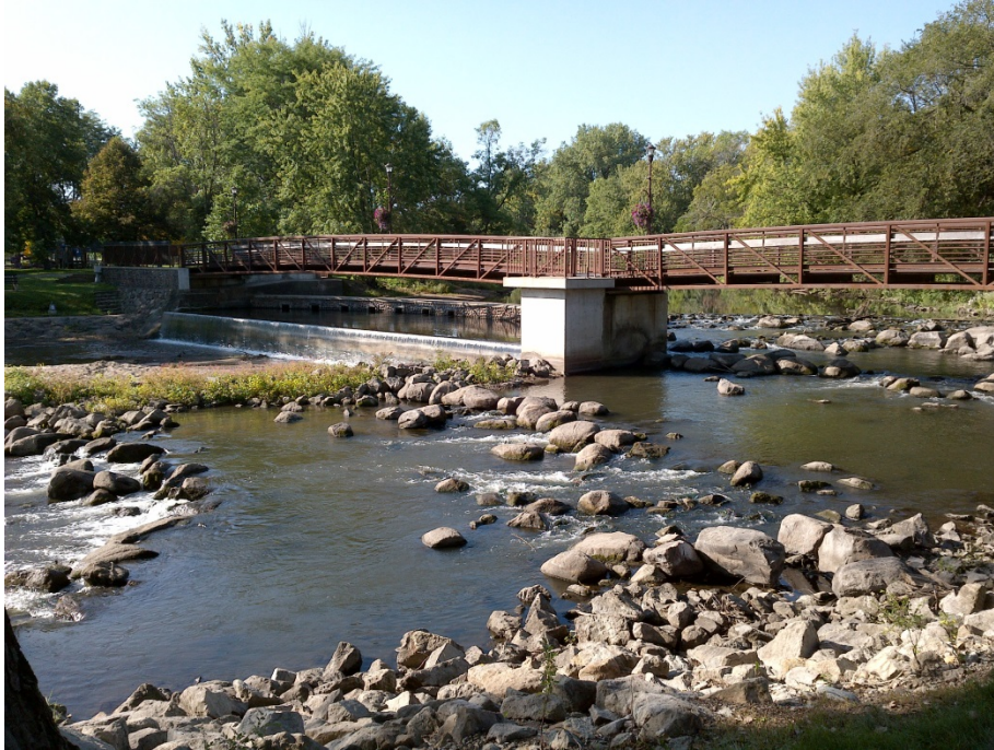
Figure 128. Morehouse Dam with fish passage step-pool system (upstream of AUID).
