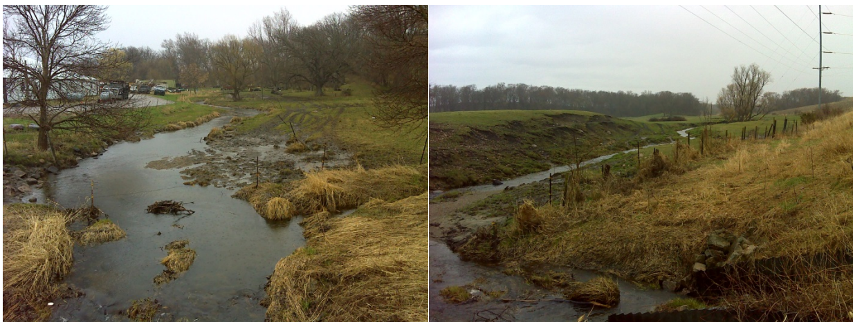
Figure 239. Upstream (left) and downstream (right) at State Highway 13, April 23, 2014
