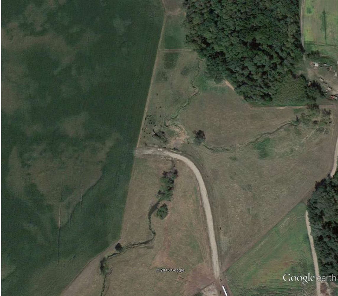
Figure 252. Field road culvert downstream of 260th St. W, SE of Morristown
