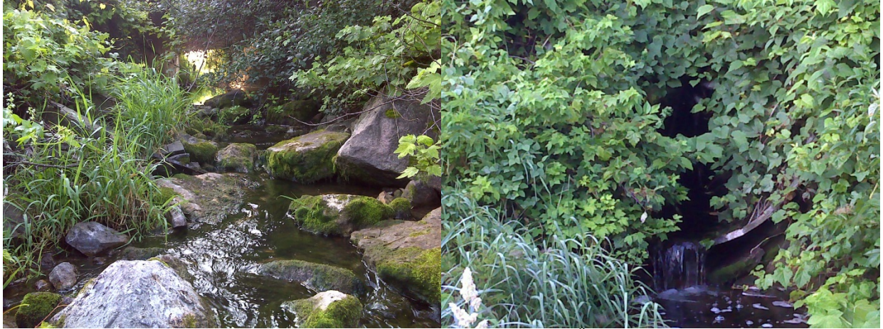
Figure 145. Passage at County Road 8 crossing (left) and perched culvert at NE 36 th Street crossing (right).
