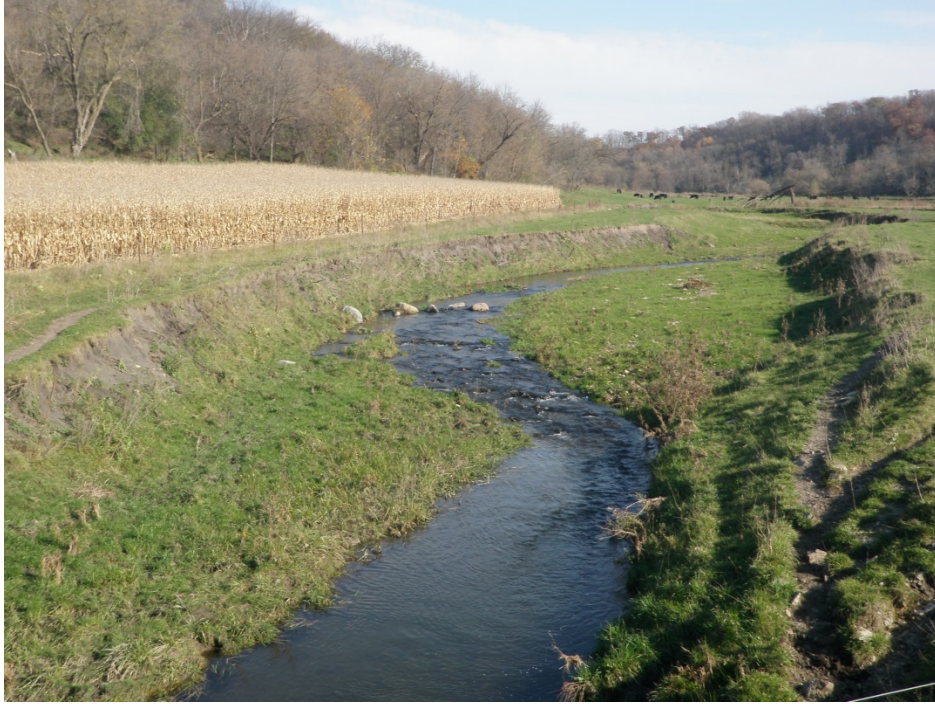
Figure 57. Eroding stream bank upstream of AUID and station 11LM027.
