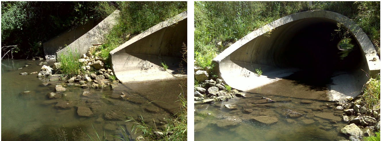
Figure 67. Stream crossing near station 11LM023 (County 14 Blvd.).
