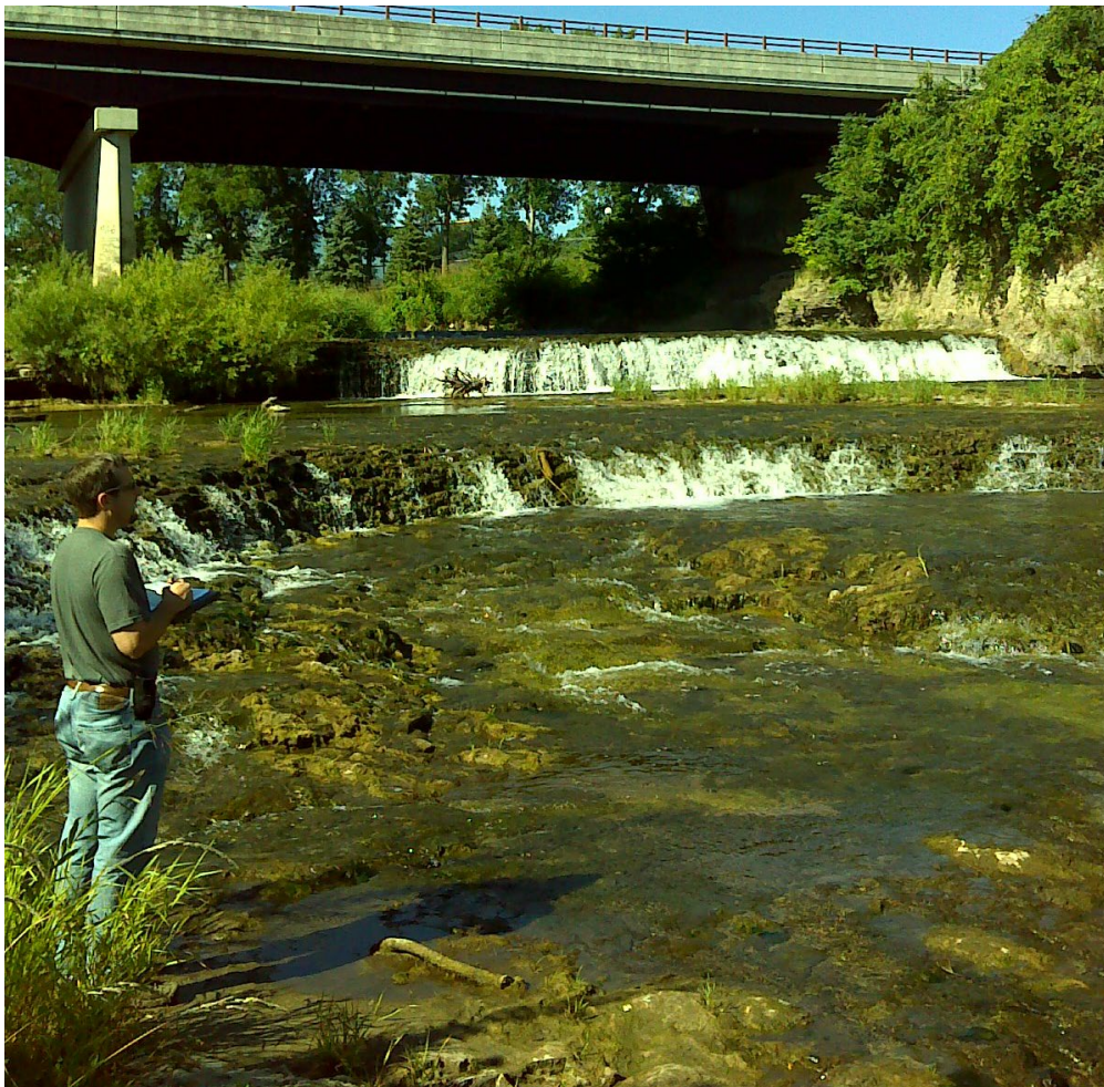
Figure 38. Migration barrier near the mouth of the Little Cannon River (Mill Street West).
