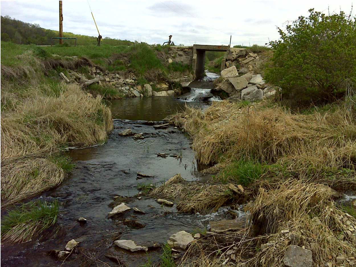
Figure 55. Fish barrier on a tributary to Butler Creek (Skunk Hollow Trail road crossing).
