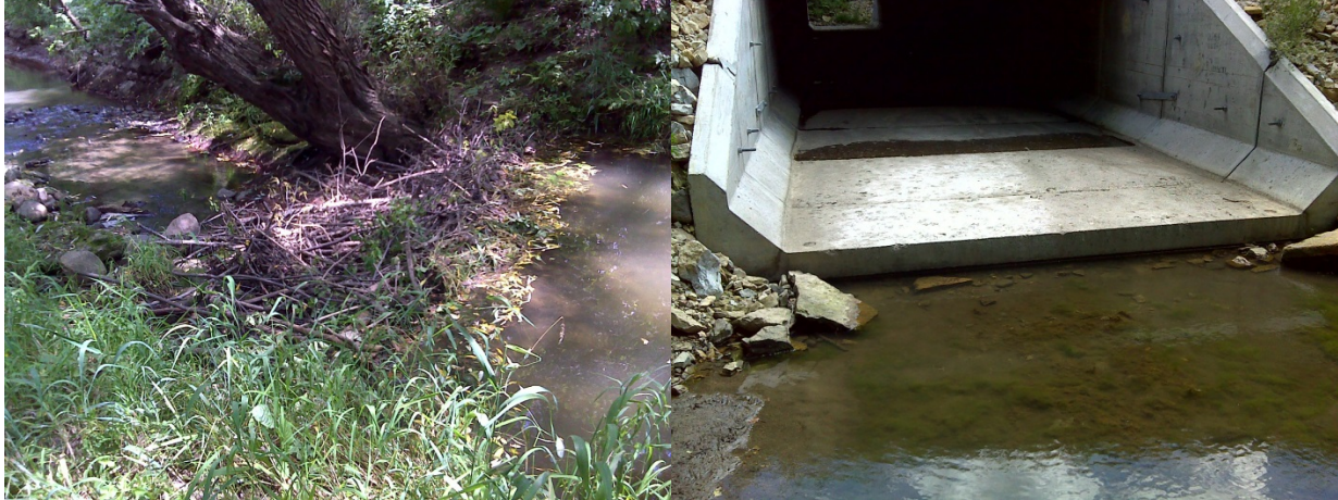
Figure 85. Beaver dam at station 11LM077 (left) and passage barrier in upstream AUID at station S001-250 (right).
