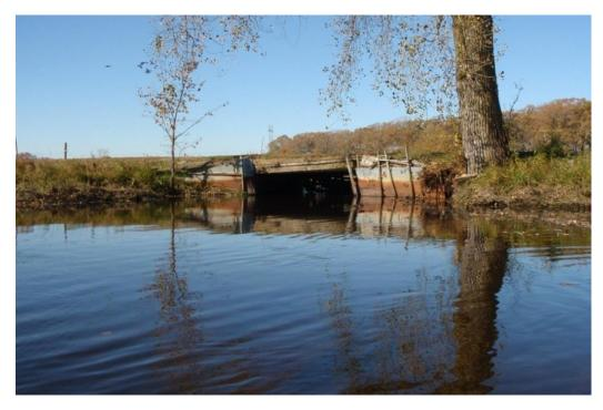
Figure 71. Undersized culvert upstream of St. Croix Trail
