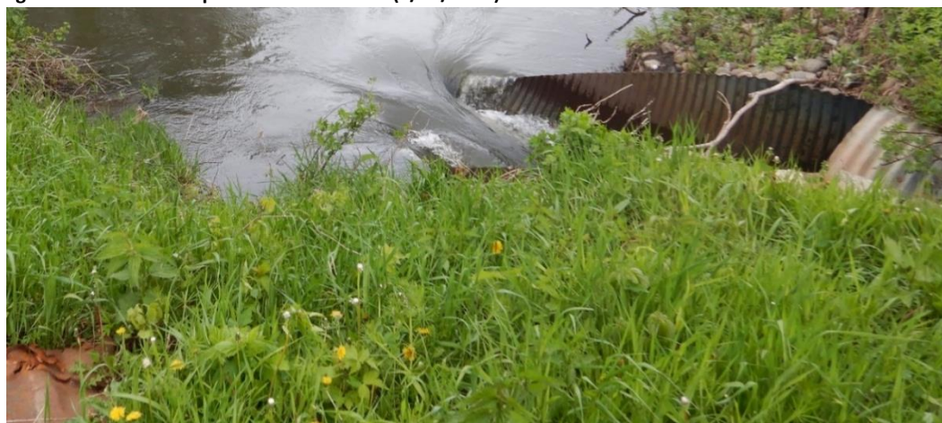
Figure 29. Culvert on upstream side of road (5/22/2019)
