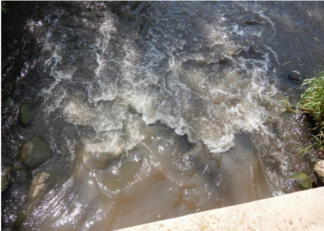
Figure 55. Culvert at site 91MN067 (6/27/19)
