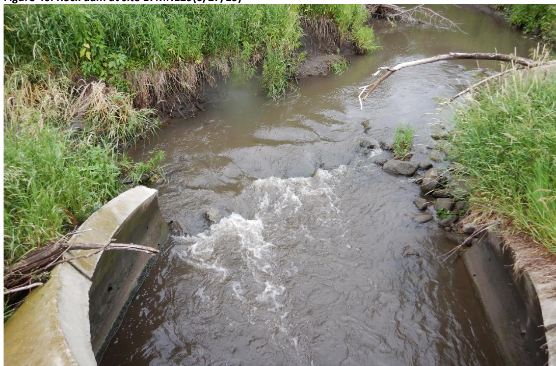
Figure 46. Rock dam at site 17MN129(6/27/19)
