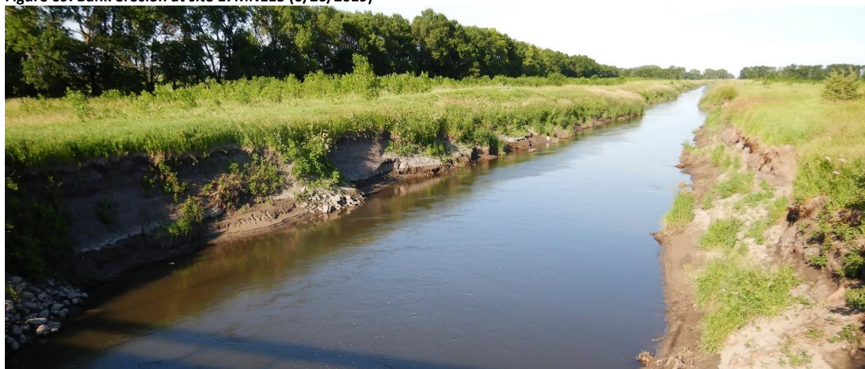
Figure 69. Bank erosion at site 17MN115 (6/26/2019)
