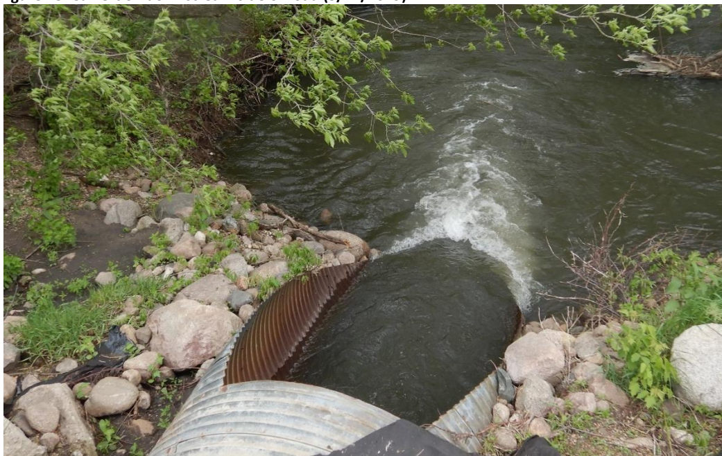
Figure 28. Culvert on downstream side of road (5/22/2019)
