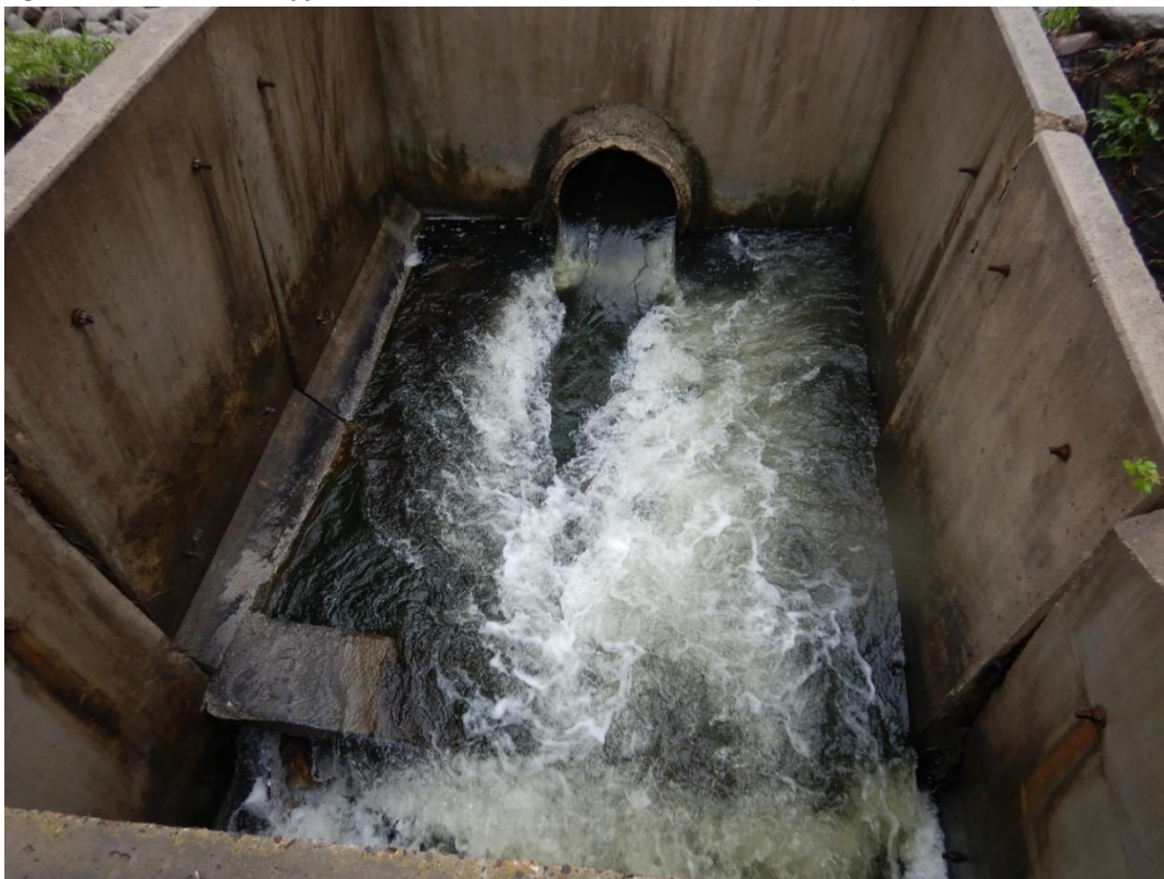
Figure 10. Culvert on the upper headwaters of the Cottonwood River (5/22/19)
