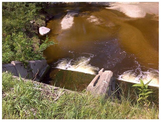
Figure 113. Morgan Creek downstream at Hwy 68, perched approximately 1 foot, August 3, 2016
