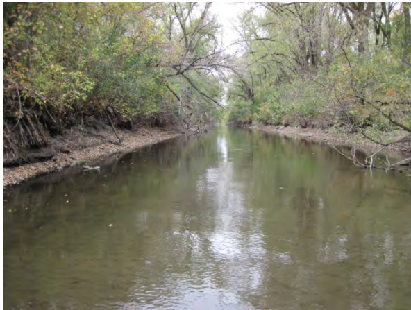
Figure 505-13 Station 03MN010 September 18, 2012, entrenched ditch with significant bank erosion.
