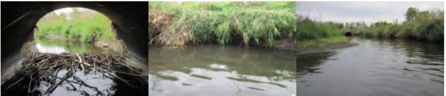
Figure 523-9 Station 09MN065 (Note beaver dam and undercut banks).
