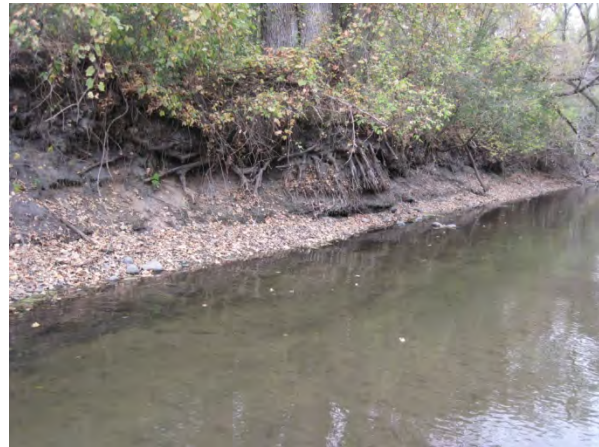
Figure 505-13 Station 03MN010 September 18, 2012, entrenched ditch with significant bank erosion.
