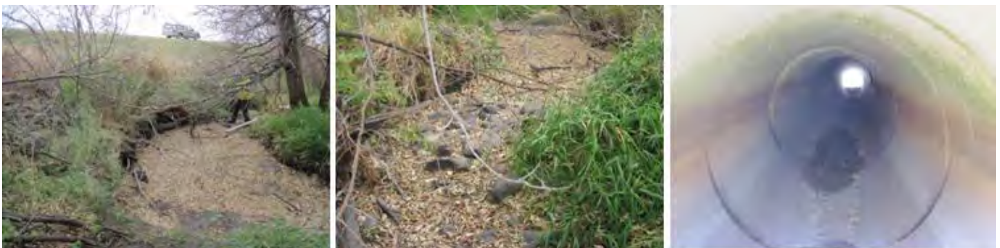
Figure 623-10 Station 03MN005 note dry channel and long dry culvert.
