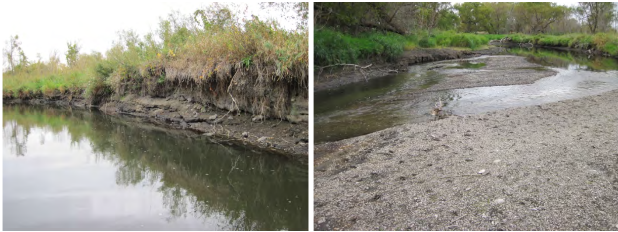
Figure 505-11 Photos of site 03MN009, note unstable banks and sandy substrate.
