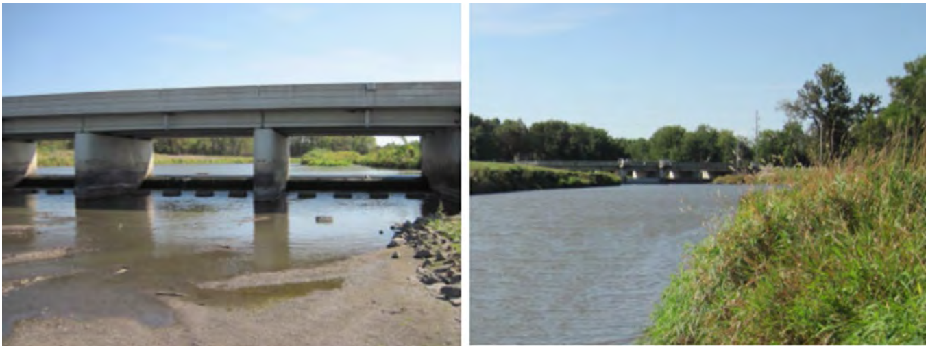
Figure 502-11 The two dams downstream of 09MN001.
