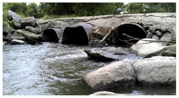
Figure 90. Undersized culvert on the West Branch Lac qui Parle River (photo credit DNR)
