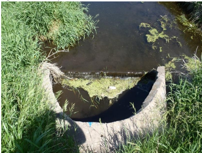
Figure 23. Culvert just downstream from bio site 15MN003
