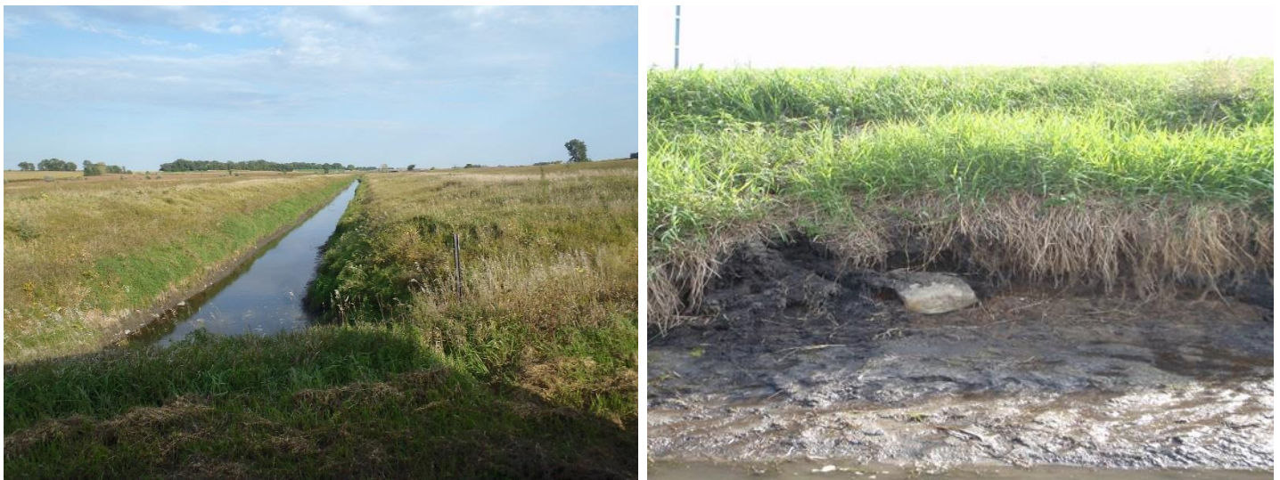
Figure 93. Photos of reach 07020001-569 showing channelization (left) as well as bank erosion and muck deposition (right)
