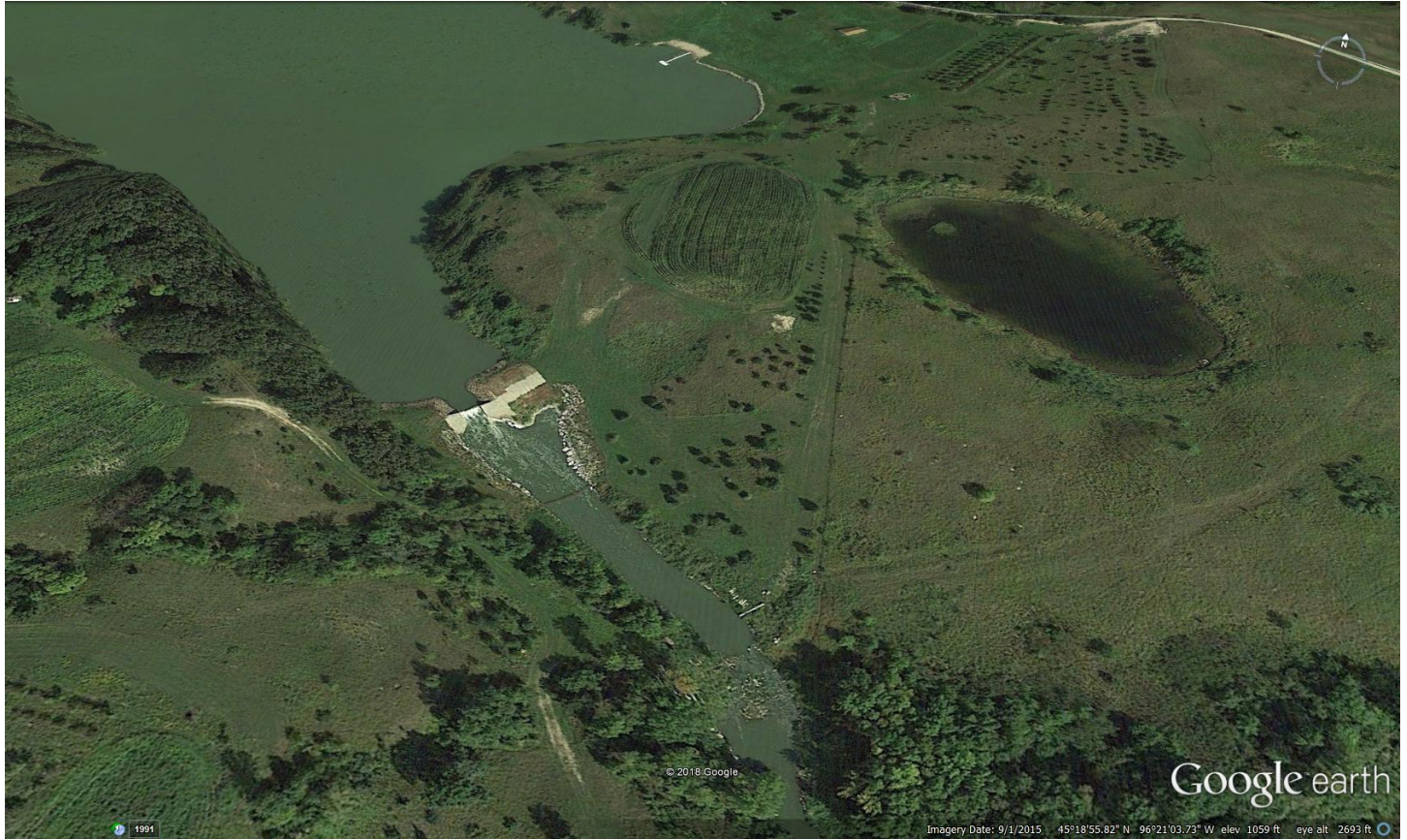
Figure 42. Google Earth image of the outlet structure that controls water levels on Long Tom Lake
