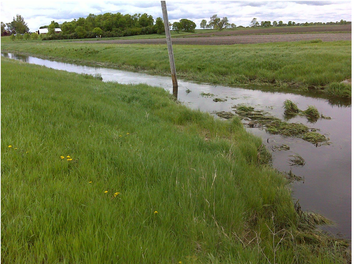
Figure 48. Photo of reach 07020001-559 showing channelization of the stream looking downstream from bio site 15MN012
