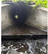
Figure 20: Perched culvert along Fish Creek.
