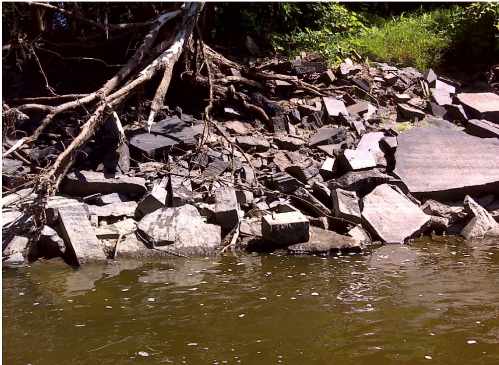
Figure 85. Dumped granite at 12UM041 (August 22, 2013)
