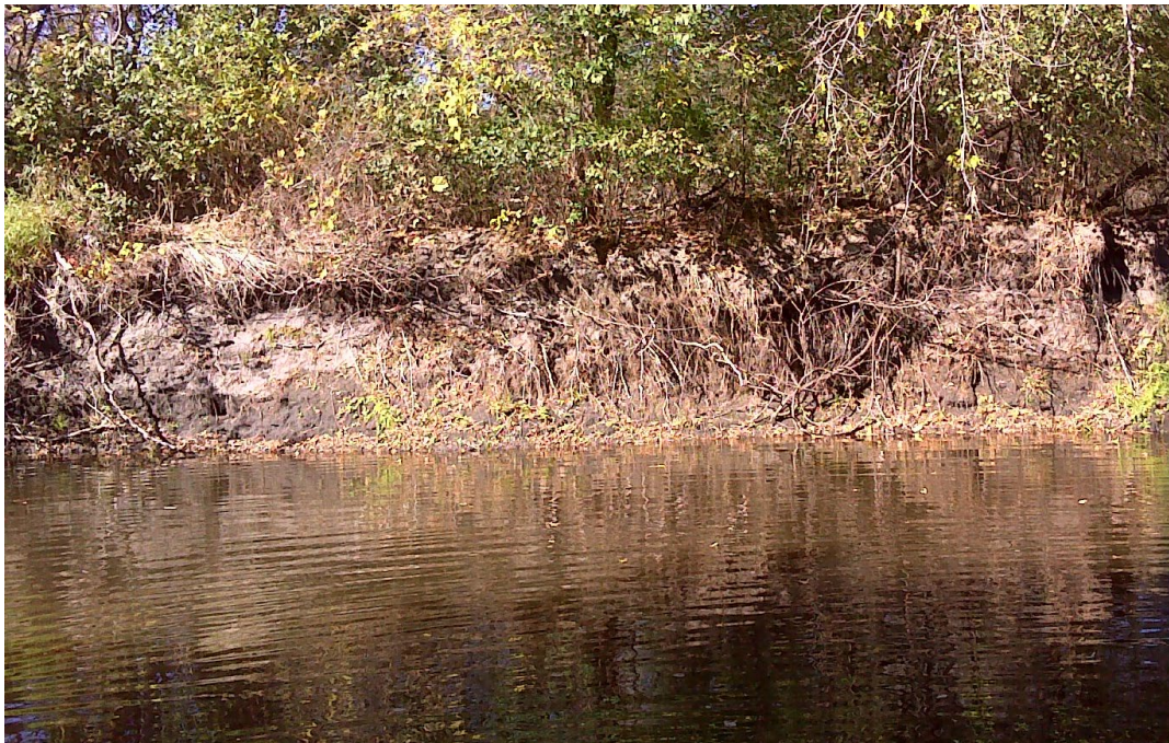
Figure 137. Eroded bank on Buffalo Creek (October 9, 2013)
