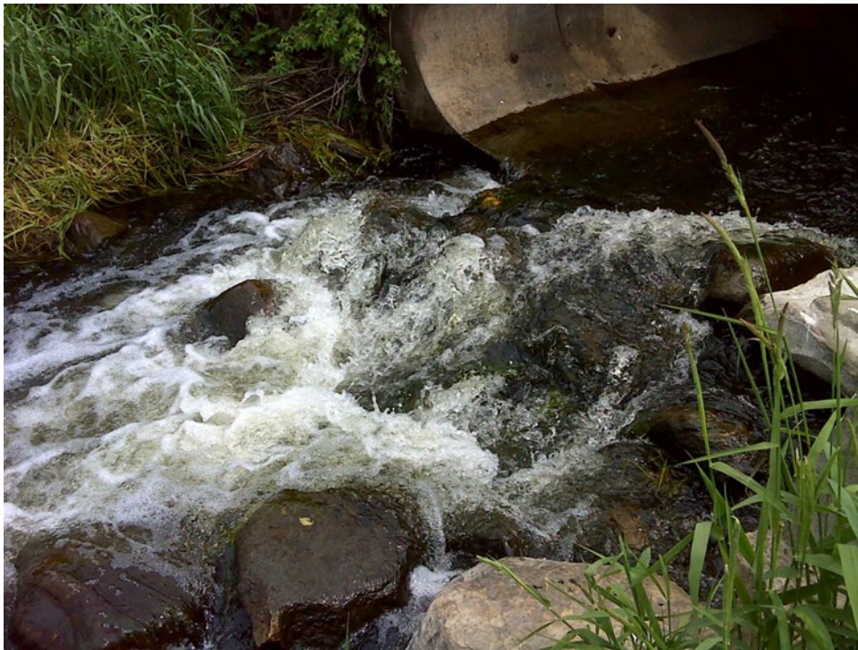
Figure 41. Culvert at station 12UM025 (June 11, 2014)
