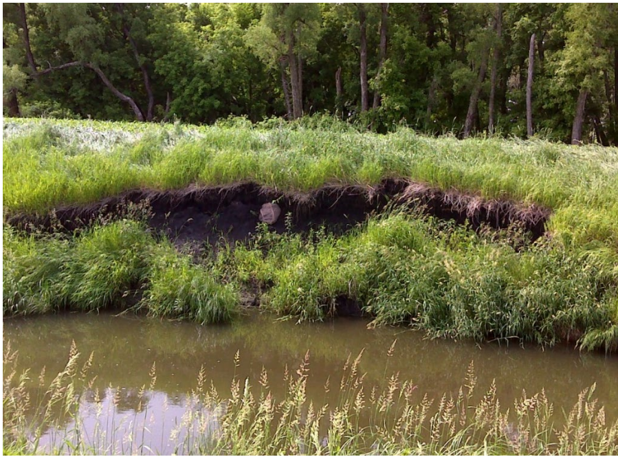
Figure 115. Erosion at 520 th (June 21, 2013)
