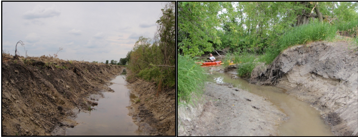
Figure 20: Photos of 2009 clean-out of a ditch flowing into the NF Crow
