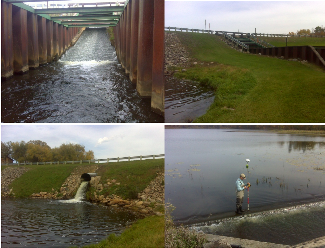
Figure 44: Photos of the dam separating the two sampling sites on Spruce Creek. The dam is acting as a fish barrier and changing the slope of the upstream channel (making the slope flatter).
