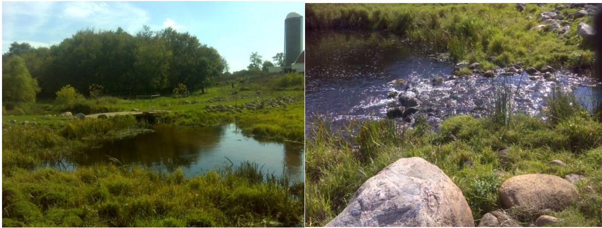
Figure 29: Photo of field crossing located downstream of 11UM013. Crossing is not causing fish passage problem; however, is causing a flattening of the stream channel slope which is causing some pool filling and aggradation.
