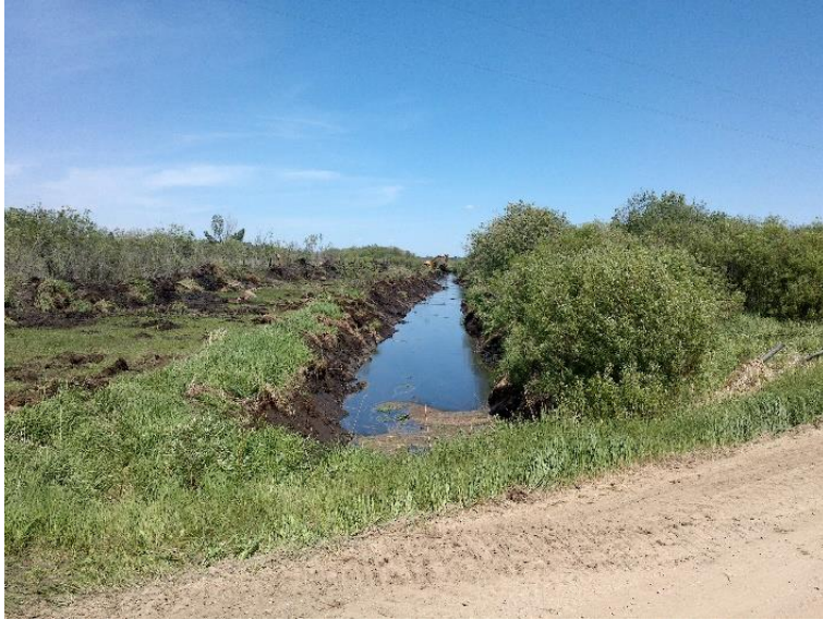
Figure 17: Tributary to Big Swamp Creek on 6/04/21, showing an almost dry channel with only 1 in of water in the channel. Channel had just been maintained in this section.
