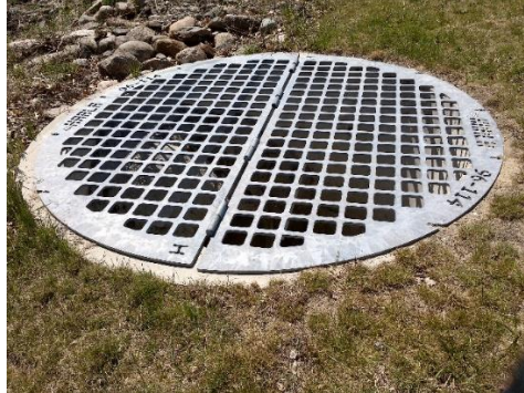
Figure 23: 5/13/2021 manhole drop structure at road crossing CR110 (CR7). Top of emergency spillway. Complete fish barrier
