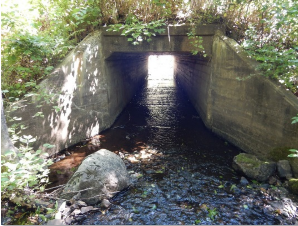
Figure 132. Captain Jacobson Creek crossing at CSAH 41
