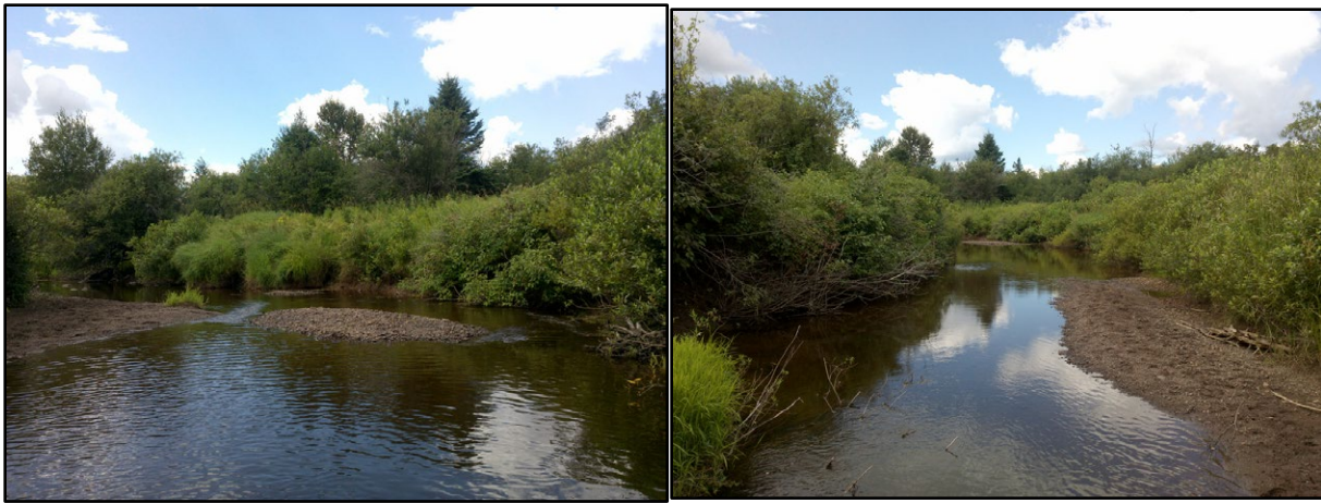
Figure 61. Mid-channel bar (left) and side bars (right) showing accelerated sediment deposition at Beaver River station 94LS005. These are indicators of channel aggradation as sediment inputs exceed transport capacity of the channel.
