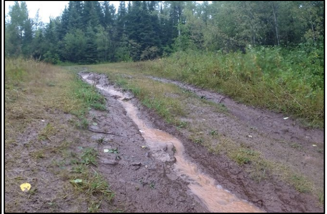
Figure 127: Surface erosion and sediment delivery at parking area at Glen Avon Falls. A parking area and hiking trail could be developed for better access and reducing sediment delivery and impacts to the riparian area.
