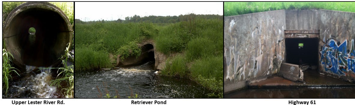
Figure 122. Examples of fish passage barriers in the Talmadge River watershed in need of restoration
