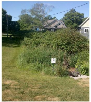
Figure 41. Rock tile inlets like this one are popular with farmers because of low installation costs, and because they can farm directly over the top of them. They are reasonably effective at removing sediment from surface runoff before entering drain tiles. This photo was taken in the NFCR Headwaters HUC-12.
