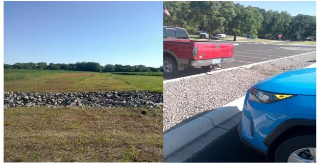
Figure 40. Infiltration basins are effective stormwater treatment if properly constructed, without compaction and with at least three feet of separation between the bottom of the basin and the seasonally high groundwater table. Photo taken in the Roseville Township, Green Lake HUC-12 070102040206.
