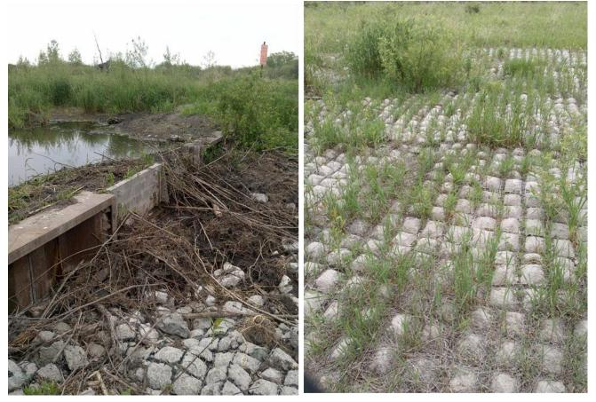
Figure 24. The Prairie Storm Project helps to settle sediment and phosphorus out of stormwater before discharging to the North Fork of the Crow River via JD 1. The intake for the water bypass had become plugged with mud due to beaver activity, causing more water to back up behind the weir than perhaps was intended. Photo taken in the Raymond Township Headwaters NFCR, HUC-12 070102040102.
