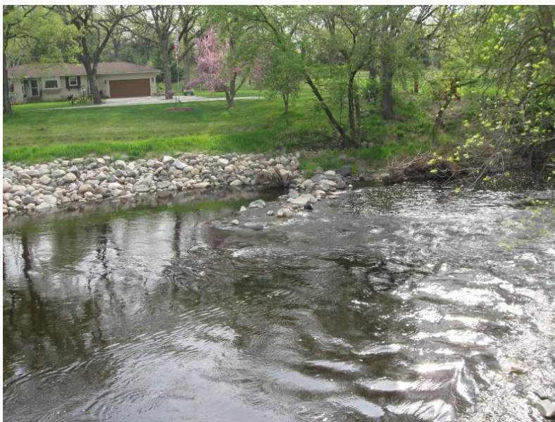
Figure 3. Post-construction site photo.
