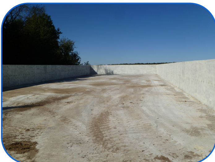
Completed Manure Stacking Slab
