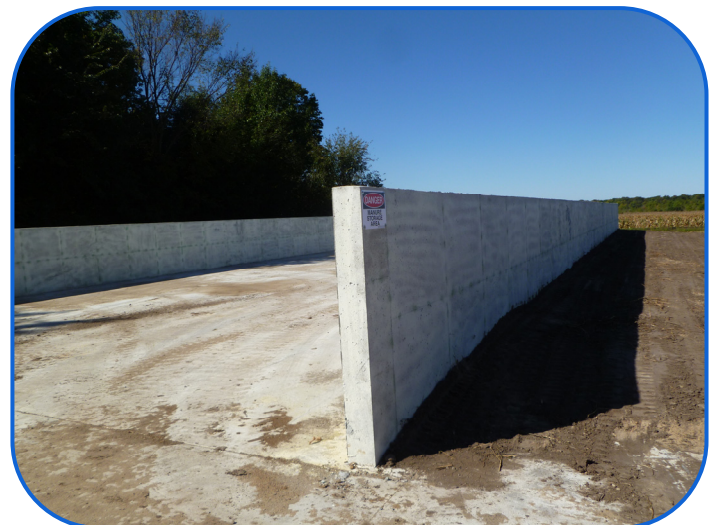
Completed Manure Stacking Slab
