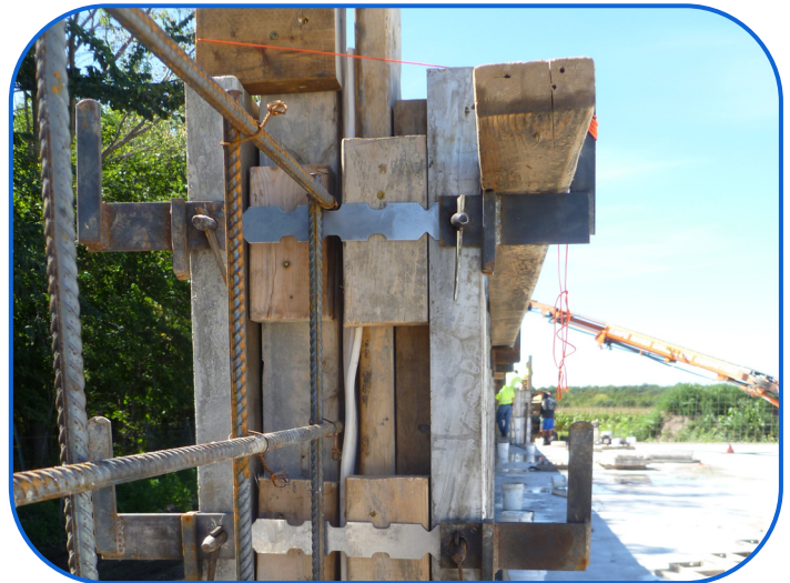
Forming of Concrete Stacking Slab Walls
