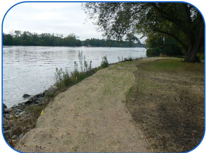
Erosion Blanket & Planting
