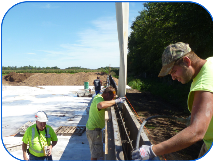
Concrete Stacking Slab Construction
