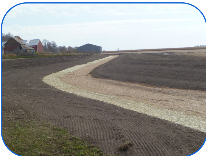
Grassed Waterway Shaped, Seeded and Erosion Blanket
