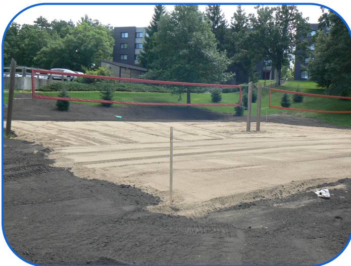
Volleyball Court Amended to a Infiltration Basin
