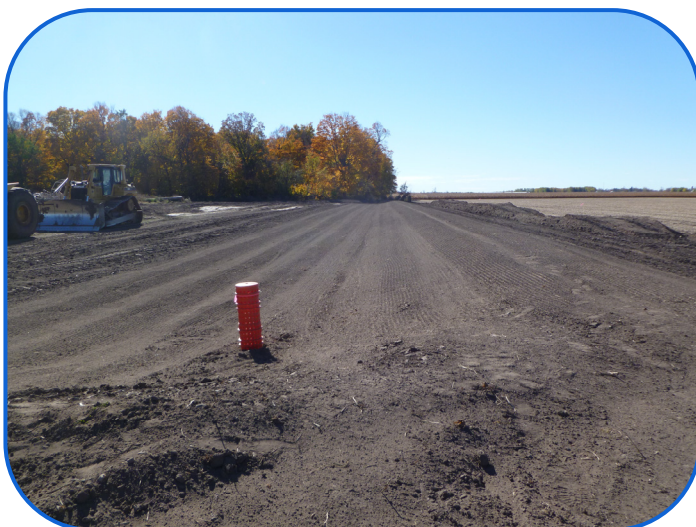
Water and Sediment Basin with Control Inlet
