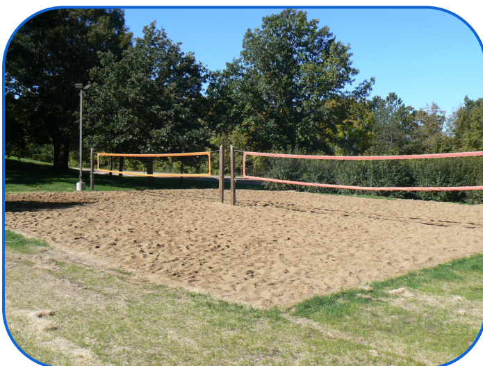
Volleyball Court Infiltrates Stormwater (See Above)
