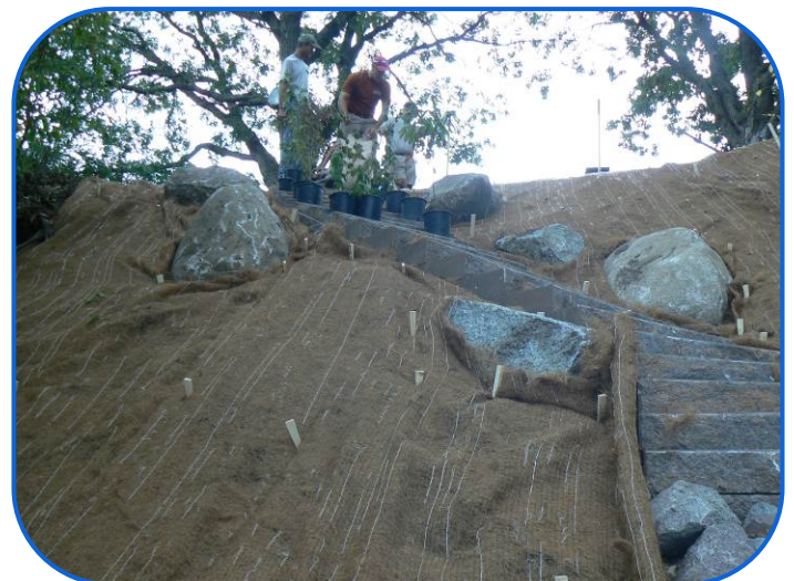
Erosion Blanket & Plant Installation
