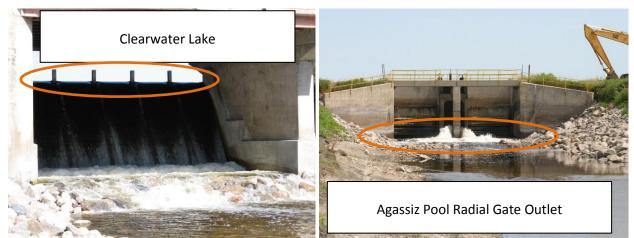
Figure 2-26. Photos showing the differences between a concrete and stop-log dam on a reservoir and the Tainter radial gates at the primary outlet of Agassiz Pool.
