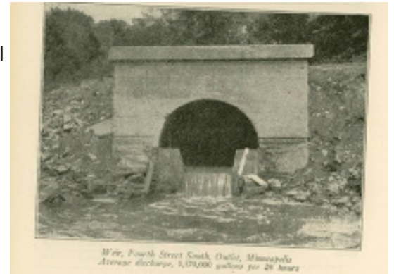
Downtown Minneapolis sewer in 1927. Over 1.5-million gallons of sewage, runoff and other waste, on average per day, flowing into the Mississippi River
