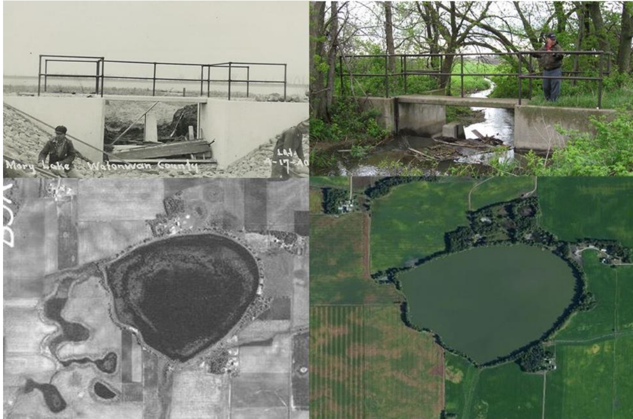
Figure 20. Outlet structure on Mary Lake in central Watonwan River watershed. Structures throughout the watershed such as this likely changed lake and stream stability, affected sediment deposition, emergent aquatic vegetation, and hydrology.
