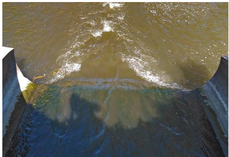
Figure 39. Culvert at the road crossing near bio site 92MN027.
