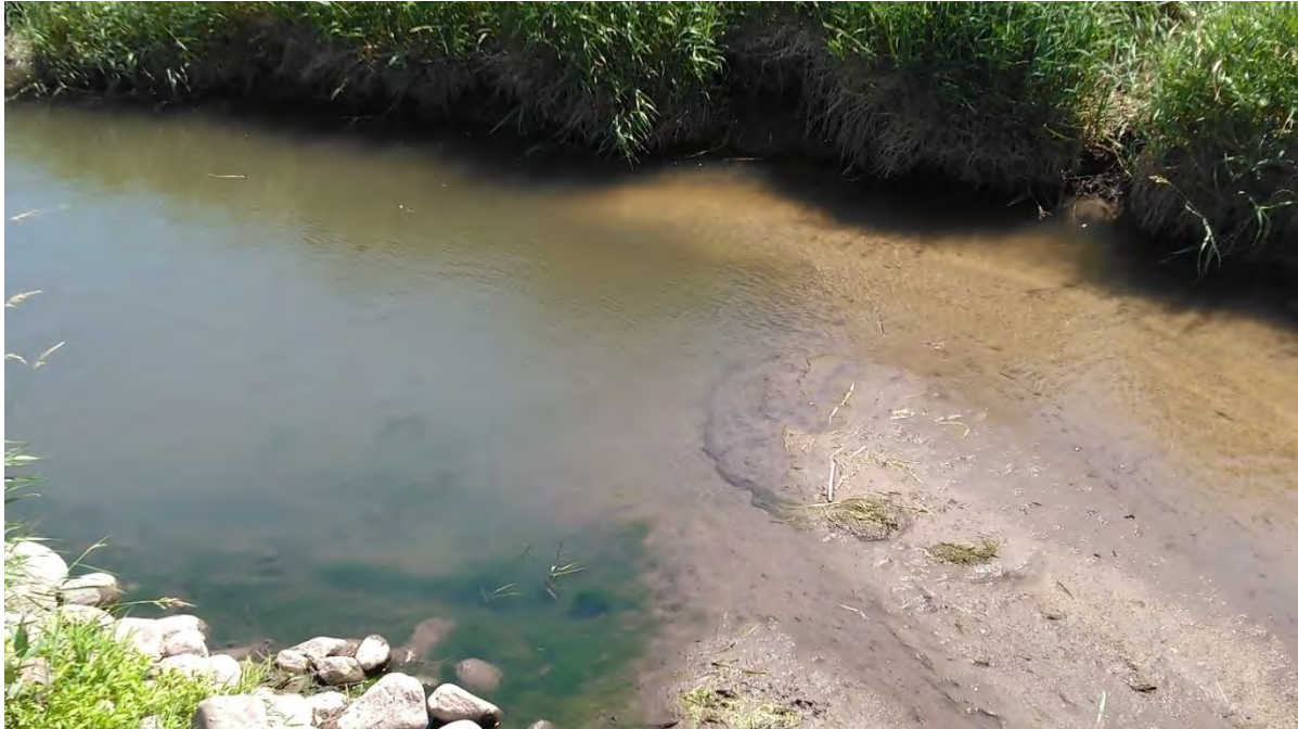
Figure 25. Photo of bio site 17MN206 showing algae growth just downstream of the road crossing right where the stream turns into a straightened ditch. There is also substantial sediment deposition on the right side of the photo.
