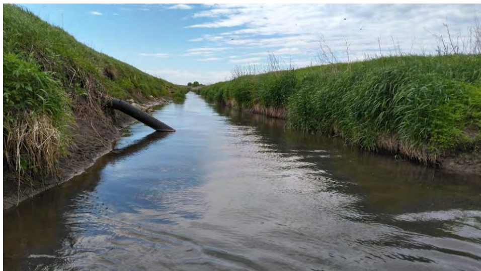
Figure 102. Photo of Bio site 17MN224. The stream channel is a straightened ditch that appears to be incised. There is very little depth variability in the stream channel.
