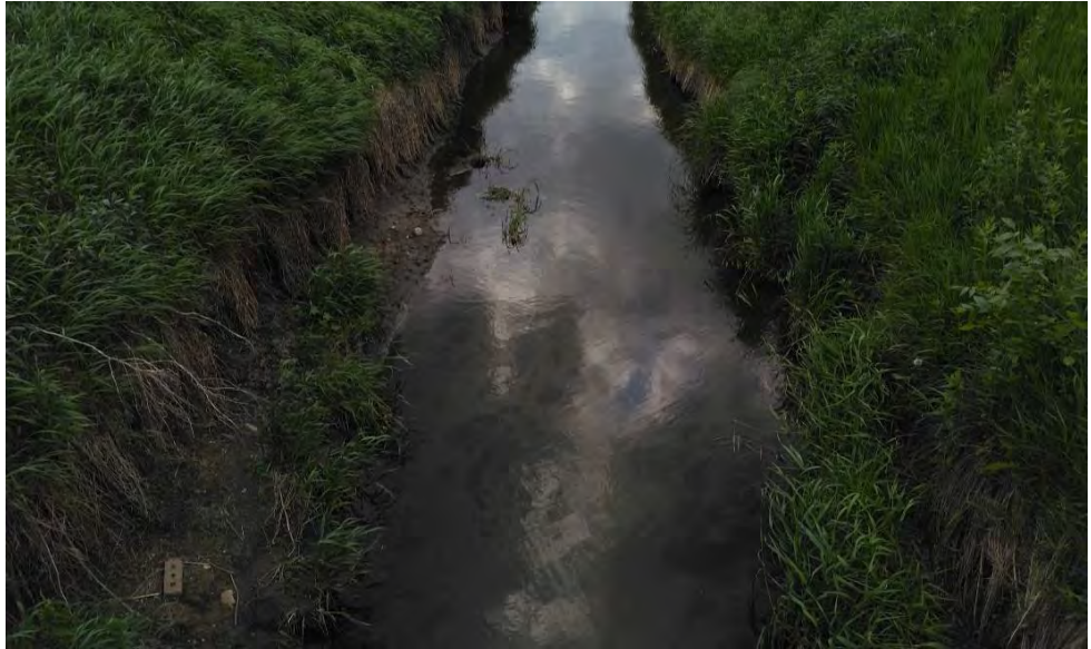
Figure 74. Photo of Bio site 17MN217 showing a straightened ditch that has been incised. There is obvious erosion along the banks.
