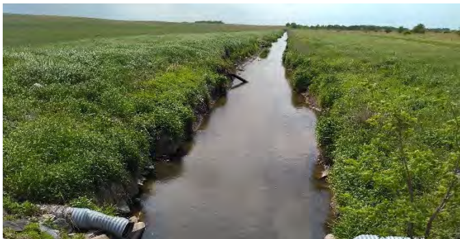
Figure 100. Photo showing a ditched stream channel at bio site 17MN224. Tile lines on the left side of the photo have been exposed due to erosion of the stream bank.
