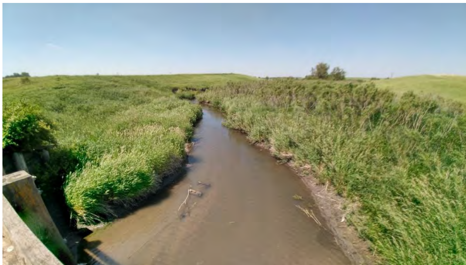
Figure 27. Photo showing the bridge crossing at bio site 17MN207 showing some sand deposition and geomorphological development. Even so, the stream appears to be widened and shallow, which provides little habitat for fish.
