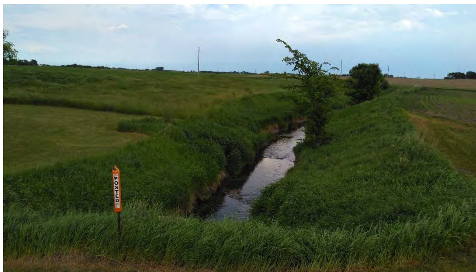
Figure 73. Photo showing the ditched stream channel at bio site 17MN217.
