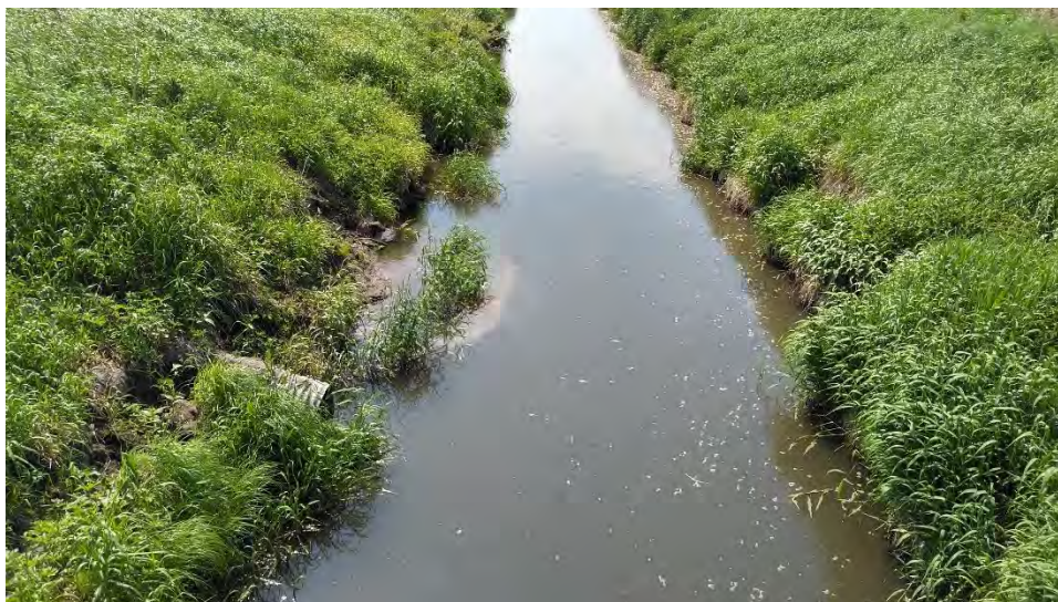
Figure 96. Photo showing upstream of road crossing near bio site 17MN227 showing a straightened ditch with unstable banks.
