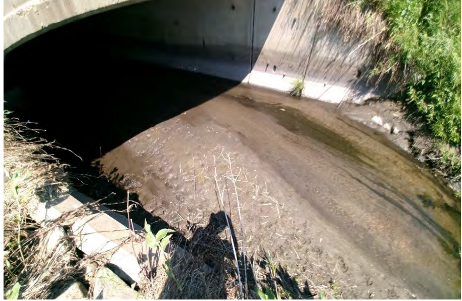
Figure 20. Bio site 17MN205 at the road crossing showing silt deposition within the channel.
