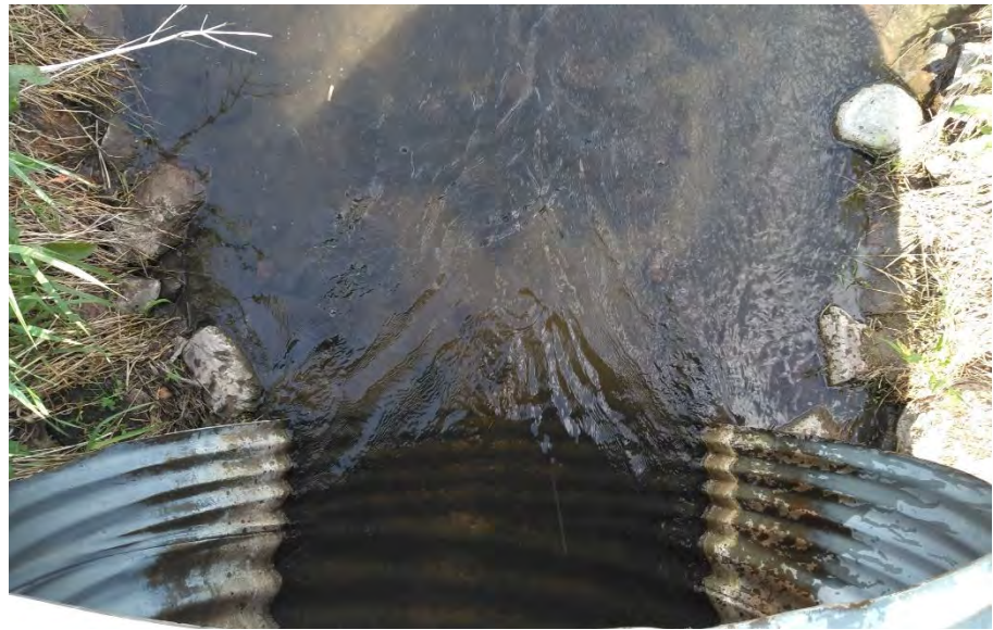
Figure 86. Photo showing the culvert near bio site 91MN040
