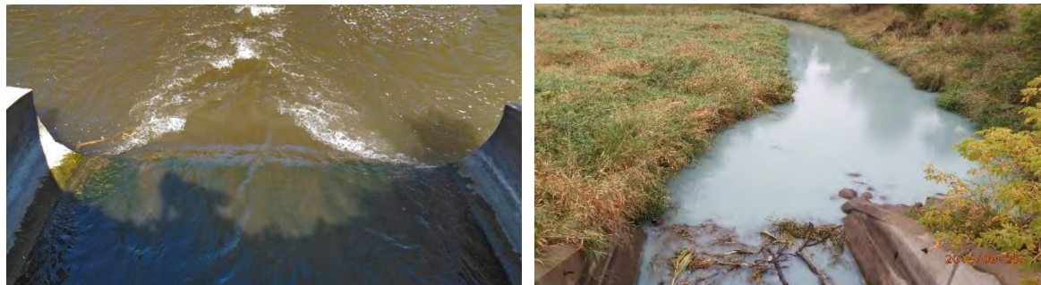
Figure 46. Photo from a field visit in 2020 showing algae growing on the culvert at the road crossing near bio site 92MN027 (left). Photo showing the creek just downstream from Coon Lake during an active fish kill (right).
