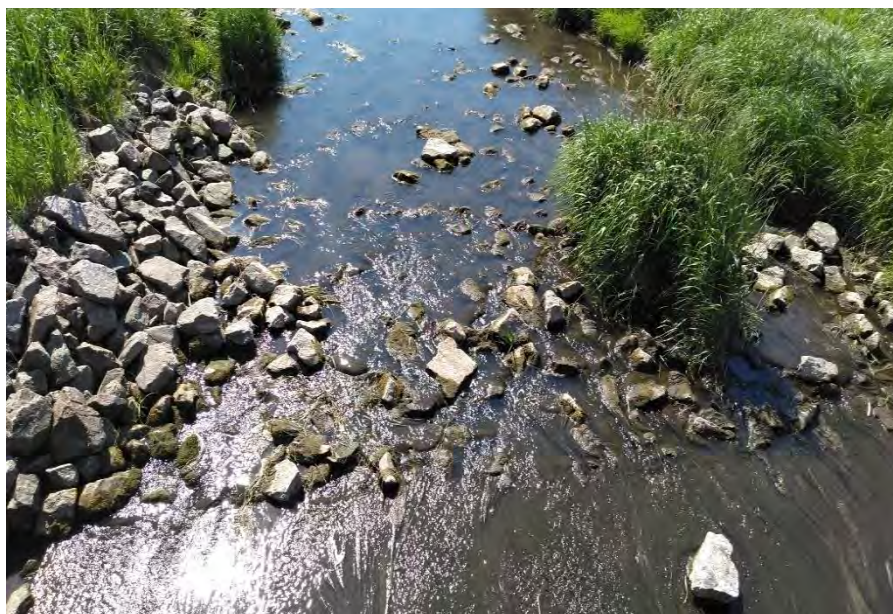
Figure 31. Artificial riffle made from cobble and boulders just upstream of the road crossing appears to be a fish barrier during low flows.
