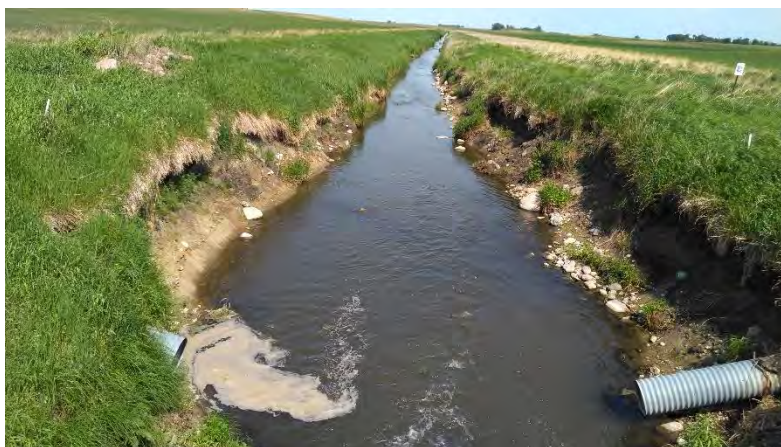
Figure 101. Photo showing the ditched stream channel near bio site 17MN227.
