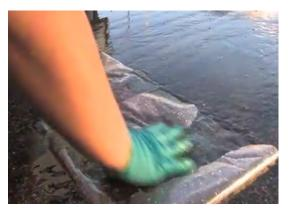
· Place the bags of sand, as shown, to help direct the stormwater flow into a narrow "channel".
