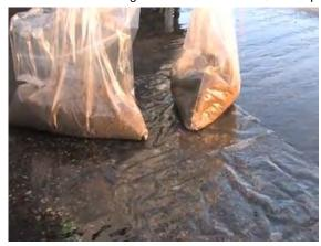
Place the straight piece of wood or metal (or the shovel handle) underneath the plastic bag on the downstream side of the bags. This should make it easier to guide the stormwater from the sand bag channel straight into your collection bag.
