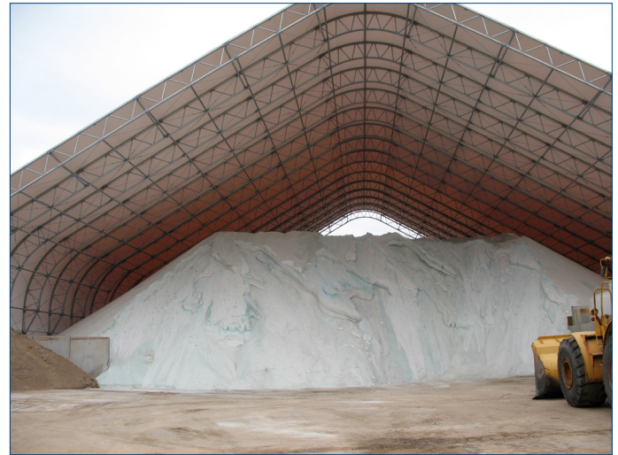
Appropriately managed salt piles should not cause contaminated stormwater runoff.
