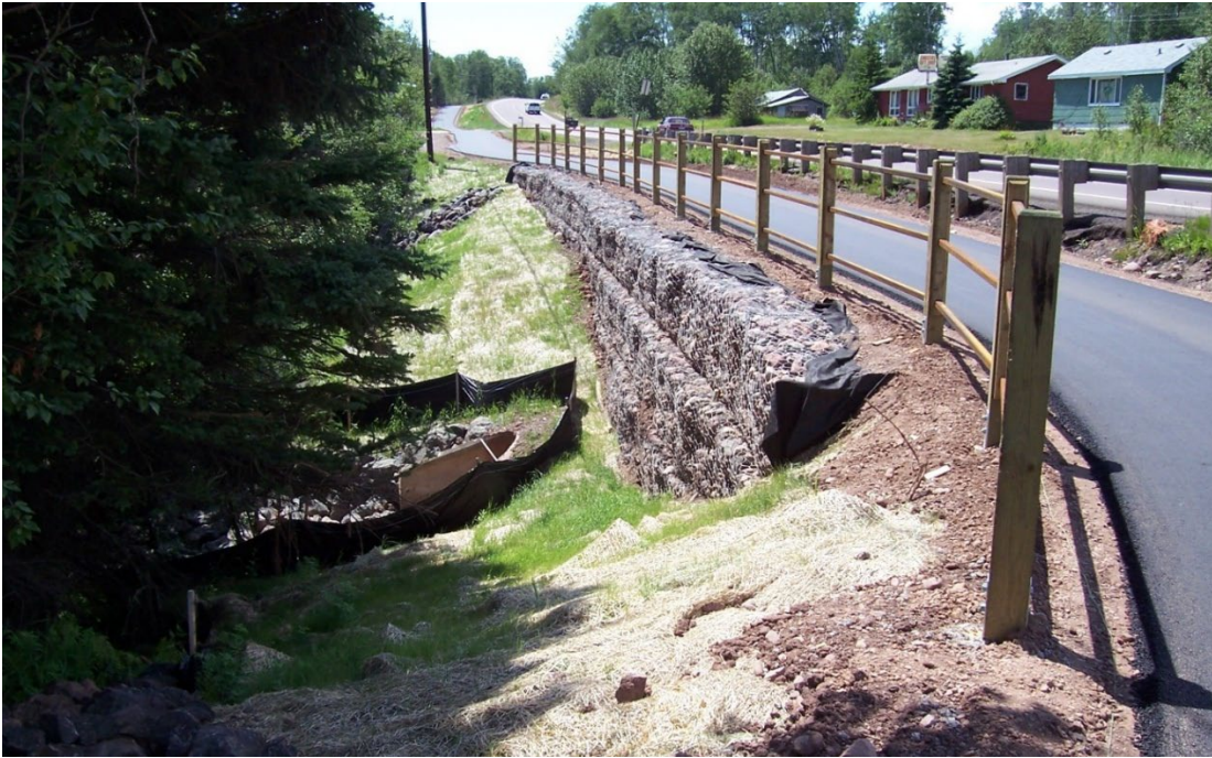
This image shows vegetative coverage of around 50% and would not be acceptable.
