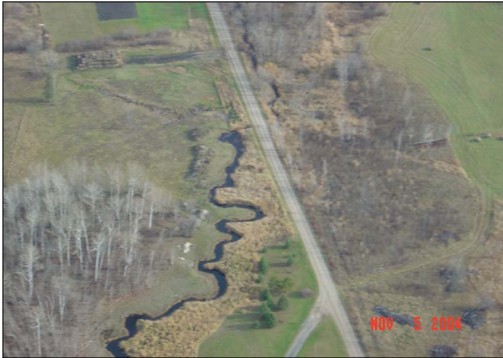
Figure 22. Channel incision and reduced sinuosity resulting from a culvert on a tributary to the Little Fork River, from 2004 over-flight.
