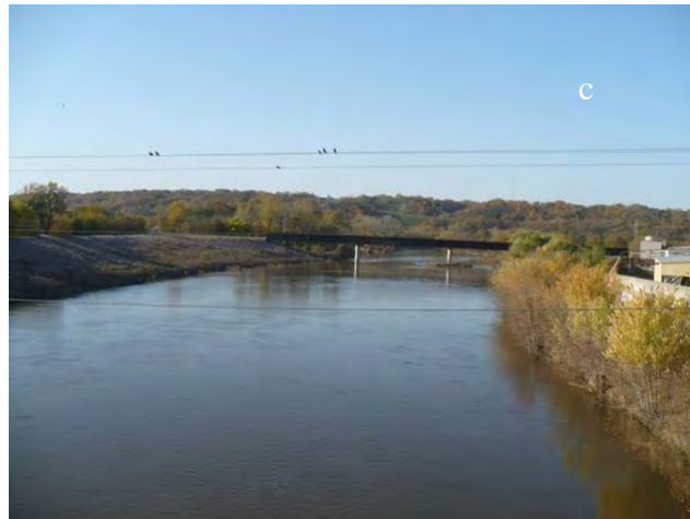
Figure 41. Levees along the Minnesota River at (a) Makato, and (b) Henderson and (c) along the Blue Earth River at LeHiller, Mankato.
