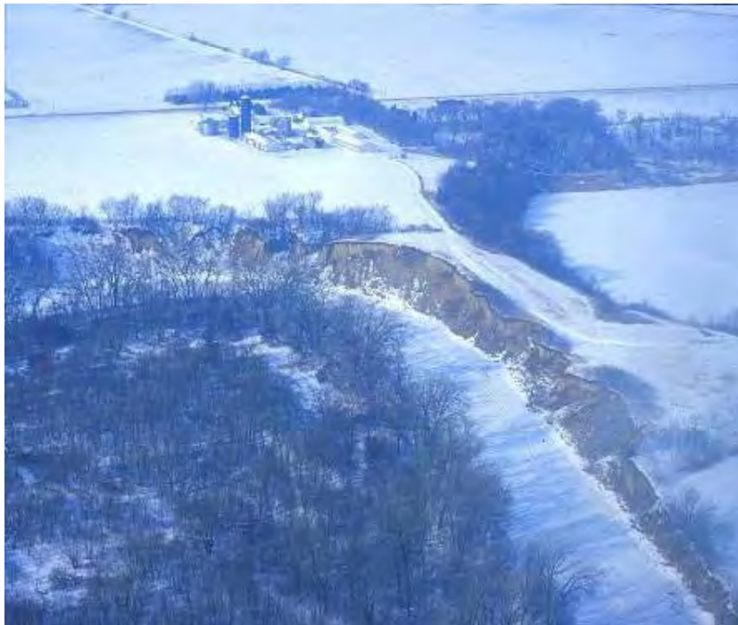
Figure 2: A picture of the sloughing banks along the Blue Earth River in Minnesota. Photograph taken by David Thoma around 2001.
