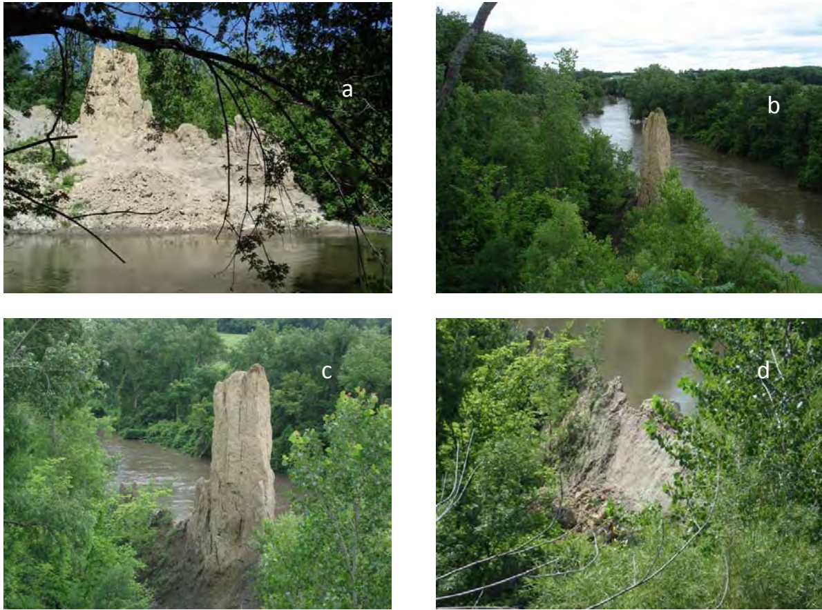
Figure 17: A series of picture showing catastrophic failure of a bank along the Blue Earth River. Dates these photographs were taken are 27 May 2010 (Fig. 17a), 28 June 2010 (Fig. 17b, c), and 5 August 2010 (Fig. 17d).
