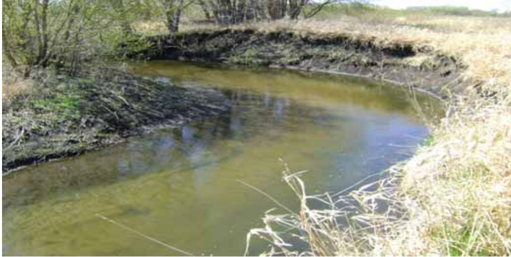
Figure 11 – Progression of streambank erosion repair with cedar trees.
