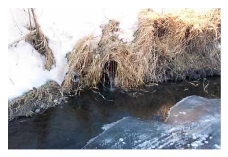
Figure 8 – Outlet of a straight pipe from a community in southeast Minnesota.
