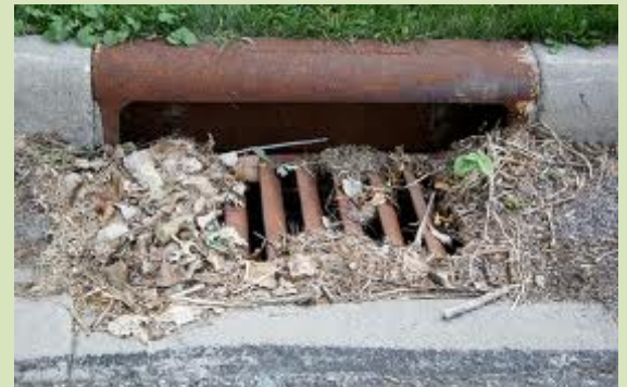
A storm drain funnels rain and snowmelt into stormwater pipes to prevent flooding. But, they also carry pollutants (like oil, deicers, and fertilizers) along with leaves and grass clippings into nearby lakes, streams, or wetlands.
