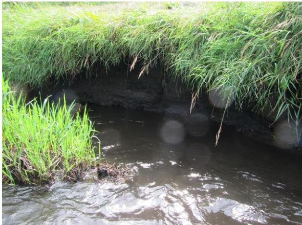
Figure 37. Bank failure at 08UM045.
