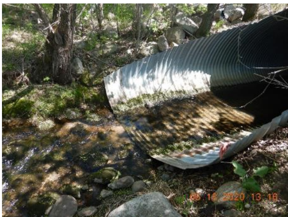
Figure 106. 260th Street culvert crossing, spring 2020.
