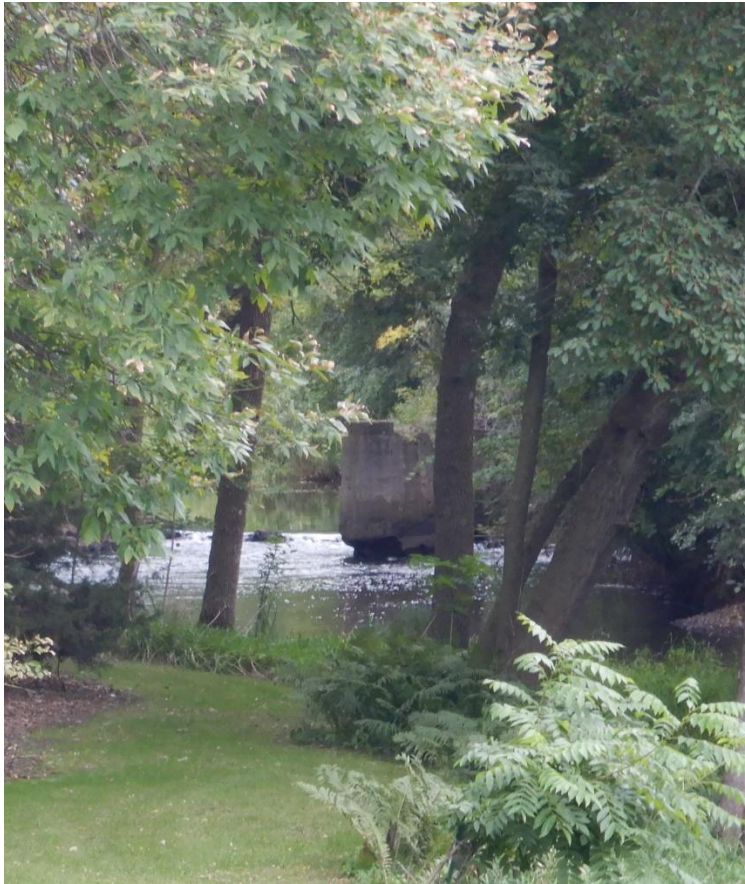
Figure 39. Old road crossing, upstream of CR 11.
