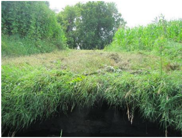
Figure 38. Bank failure at 08UM045, with crop field planted to stream edge.
