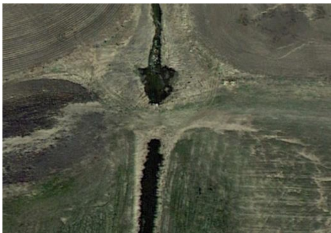
Figure 52. Field crossing with poorly placed culvert on Unnamed Creek.
