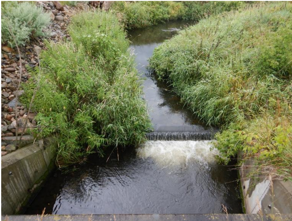
Figure 89. Weir structure upstream of the 343rd culvert crossing on Stony Creek.
