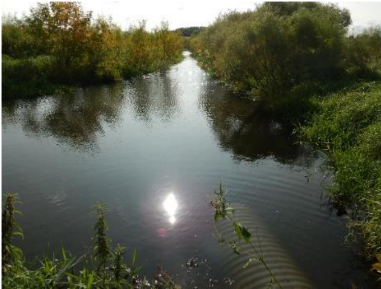
Figure 88. High flow conditions at the culvert crossing near 13UM172.
