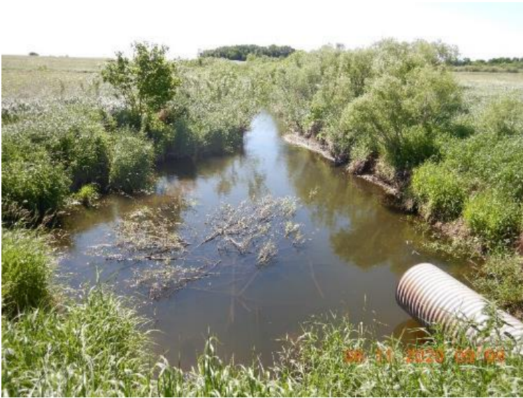
Figure 87. Low flow conditions at the culvert crossing near 13UM172.
