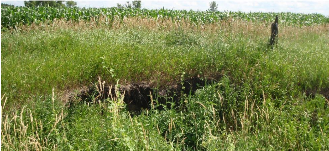
Figure 49. Bank instability at Unnamed Creek in 2008.
