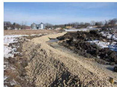
Segner Pond's limestone filter dike will remove additional phosphorus from water before it enters Cedar Lake.
