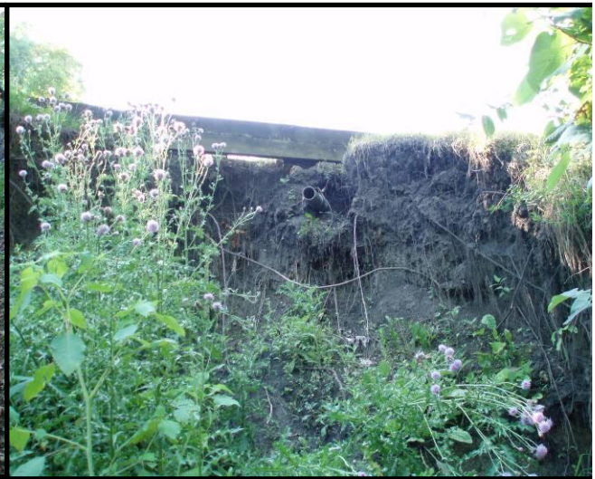
Figure 4.37 Pipe outlet from golf course (Site 18)
