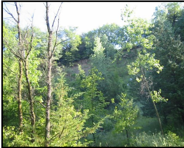
Figure 4.22 Large slope failure with Revegetated lower bank (Site 11)
