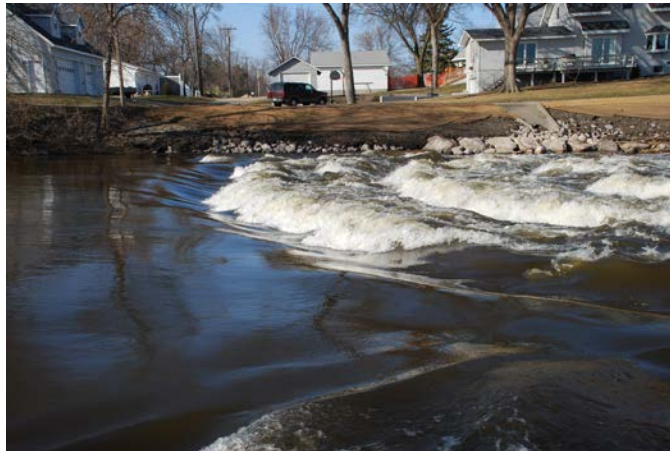
Figure 2.3 Photo Dawson Dam (tLqP-29.0 WB1.6) received by email on March 29, 2010.
