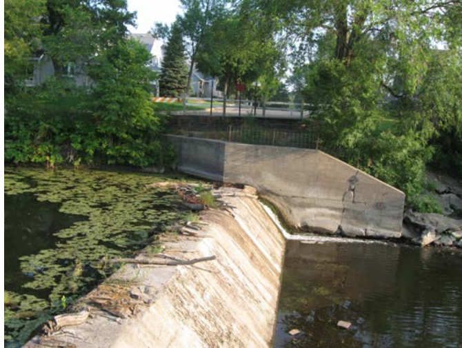
Figure 2.2 Photo Dawson Dam (tLqP-29.0 WB1.6) September 10, 2009 at 8:40am.
