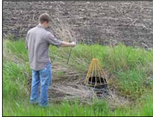
An open tile intake along the edge of an agricultural field.
