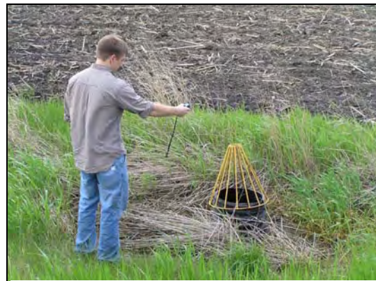
An open tile intake along the edge of an agricultural field.
