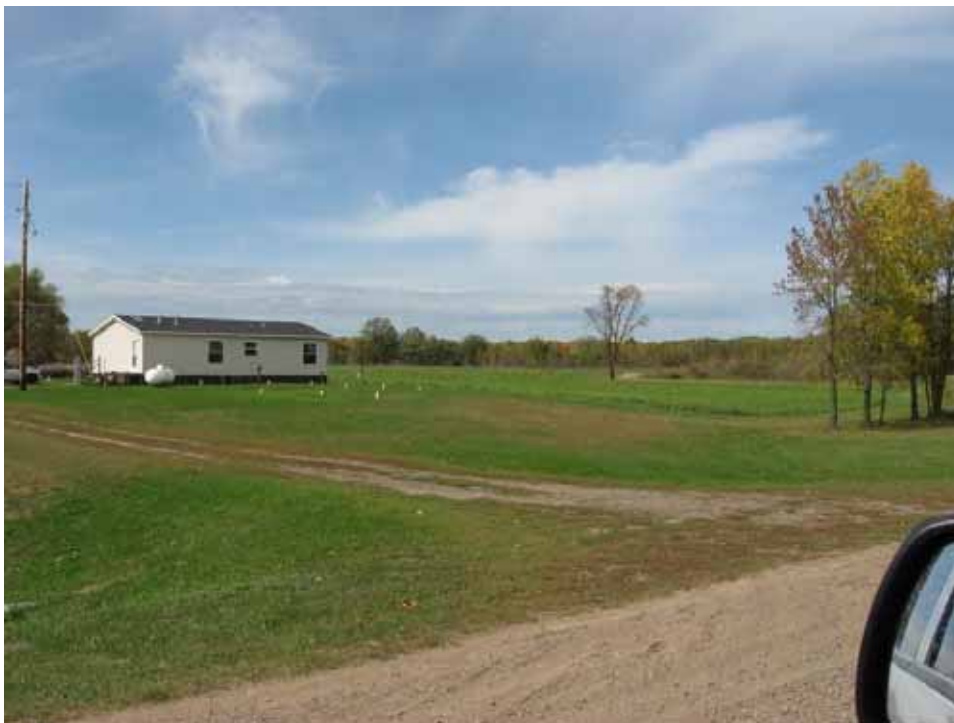
An example of a mound septic system (note the white pipes in the foreground of the house) within 100 feet of the Groundhouse. This site is just upstream of the Hwy 10 crossing.
