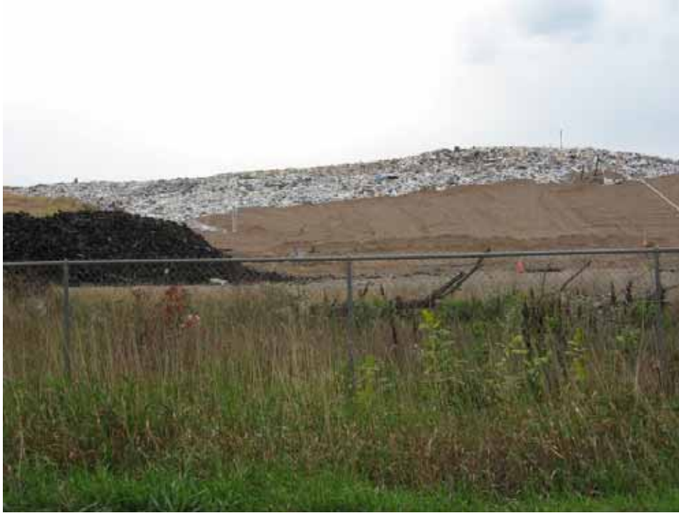
Solid waste in the landfill left uncovered after the facility closed for the day.
