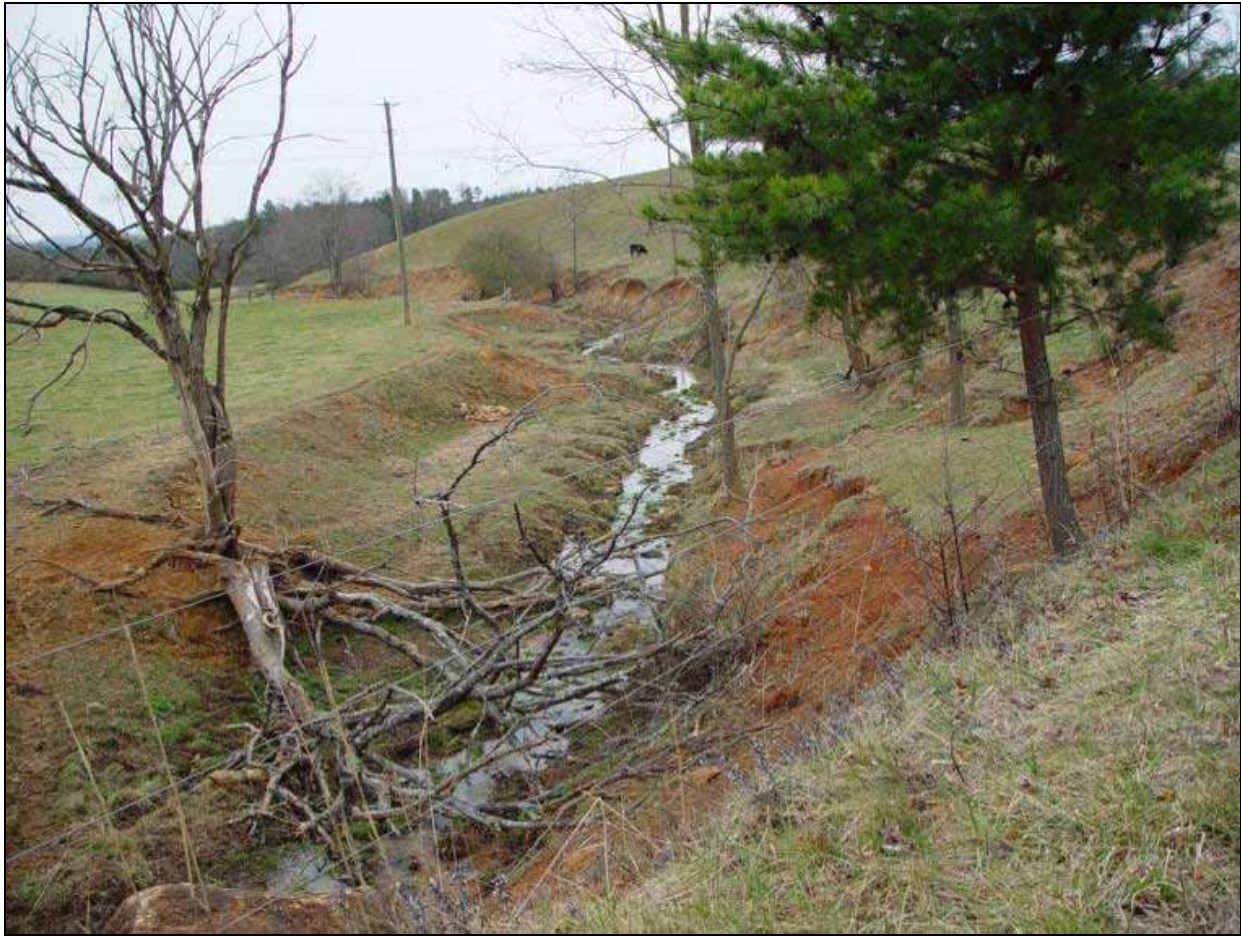
Figure 14. Typical Stream Bank Erosion in Pastures with Cattle Access to Stream
