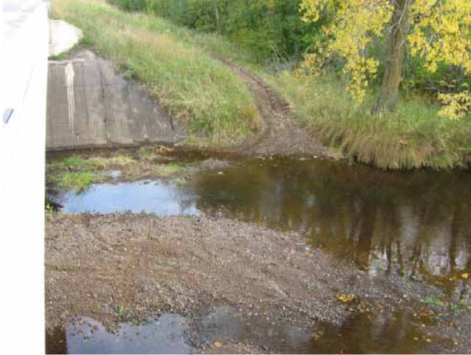
Downstream view of the Groundhouse from the Hwy 47 crossing. Where the channel is overly wide due to the road crossing, a gravel mid-channel bar has formed. Note the ATV access trail and tire tracks on the bar.
