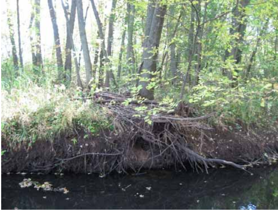
Fluvially transported woody debris along the right bank. This debris indicates that hydraulic stresses, particularly on the toe of the streambank are sufficient to erode and transport streambank material.
