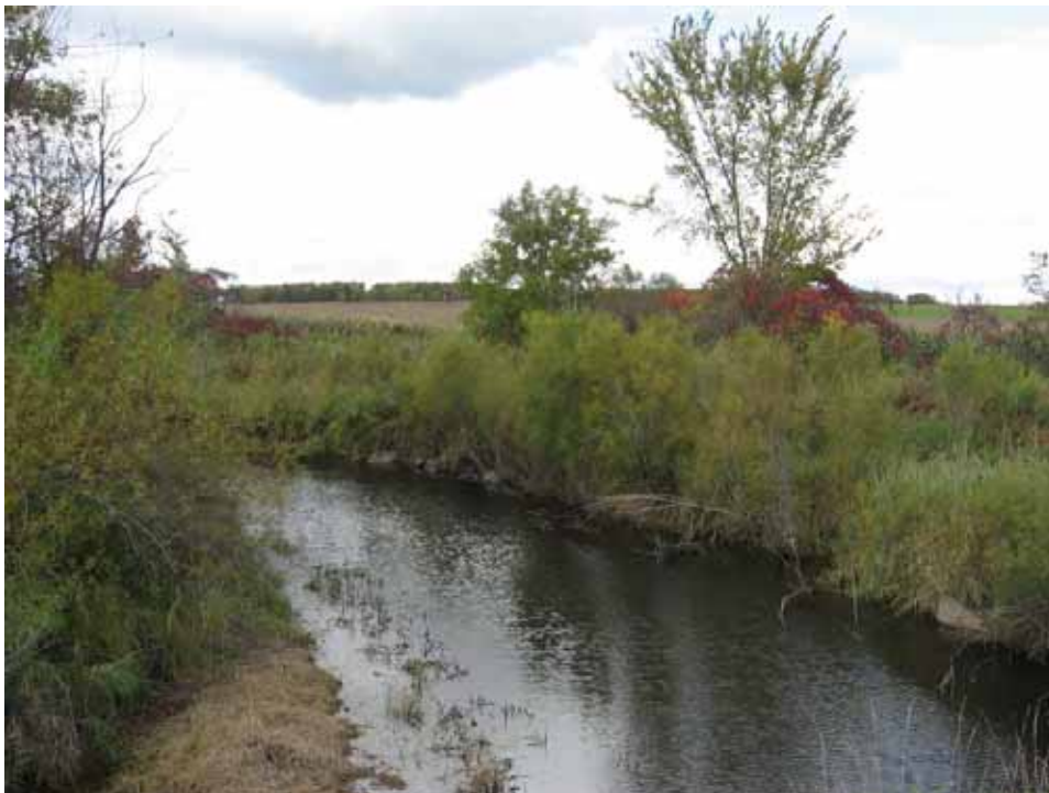
Upstream view of the South Fork at the CR-4 crossing. Boulders or possibly rip rap placed at the toe of the streambank along with the willows effectively control erosion along the toe of the bank. Row crop (corn) is visible in the background of the photo.
