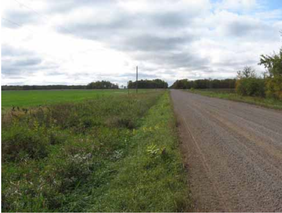
Upstream view of drainage ditch along CR-50 (facing south). Due to the well maintained road surface and the vegetation in the ditch, most eroded sediment is likely trapped in the ditch before being transported to the river.
