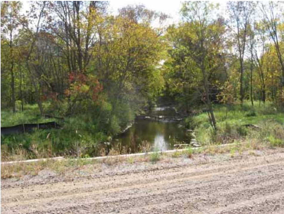
Upstream view of CR-49 crossing of the South Fork. The prismatic shape still indicates historic channelization of this reach.
