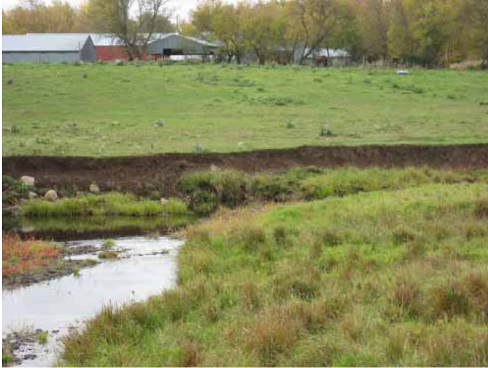
Another close-up view of the streambank erosion. This reach of the river is located in glacial outwash sands that afford little resistance to hydraulic stresses – particularly when no woody vegetation is present and livestock can trample the banks.
