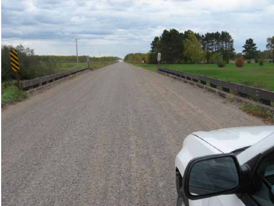
View facing south along Hwy 10 at the Groundhouse crossing. Note the well maintained condition of the road surface. The grade of the road is sloping away from the River.
