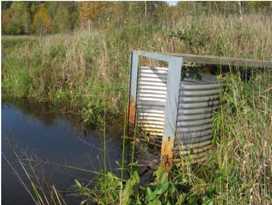
Another view of the outlet structure.
