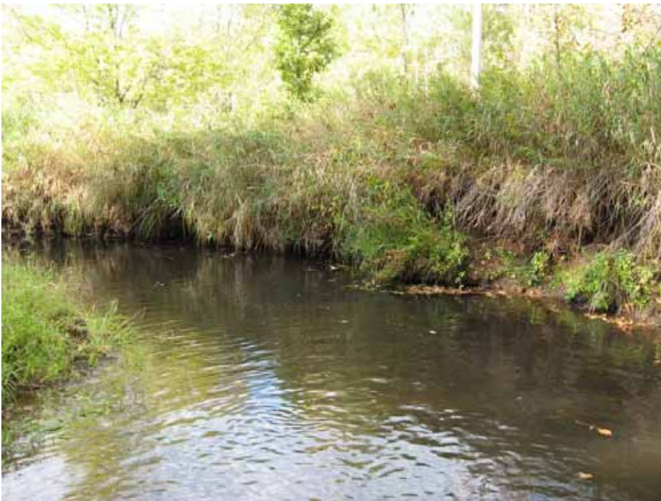
Downstream view of streambank shown in the previous photo. Scour at the toe of the bank leads to undercutting and slumping of the upper bank. This was the primary mechanism for streambank sediment input observed along this reach of the Groundhouse River.
