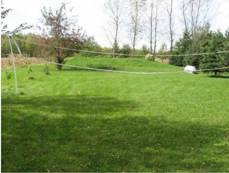
Example of mound-type septic systems commonly used in the watershed. This mound was located approximately 250-feet from the Groundhouse River (other mounds were observed closer).
