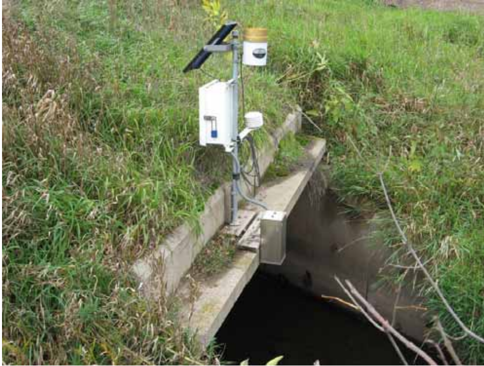
Rain gage and acoustic Doppler velocity (ADV) meter on the left of three culverts under the 140 th Street crossing of the Groundhouse. No information was posted as to the owners of the equipment.
