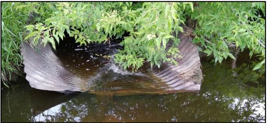
Figure 4-37. Damaged culvert along the Poplar River (AUID 518) at 310th Avenue Southeast
